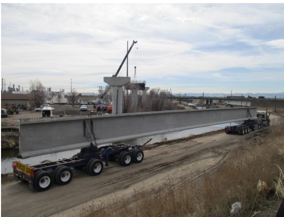
Fig. 4 Skyway Bridge Girder Being Delivered to the Site
