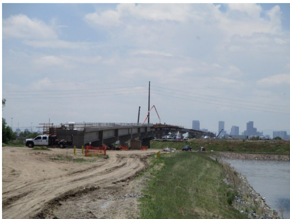
Fig. 2 North Approach of the Skyway Bridge during Construction
