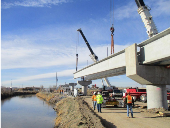
Fig. 5 Skyway Bridge Girders Being Erected at the Site
