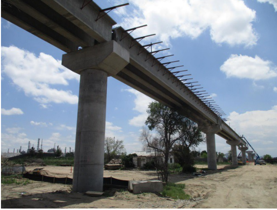
Fig. 3 Skyway Bridge Spans Under Construction
