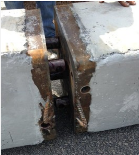
122 123 Fig. 4 – Splice connection during alignment (left) and installation of locking pins (right) 124
