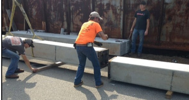
119 120 Fig. 3 - Pile supported by crane and wood dunnage 121
