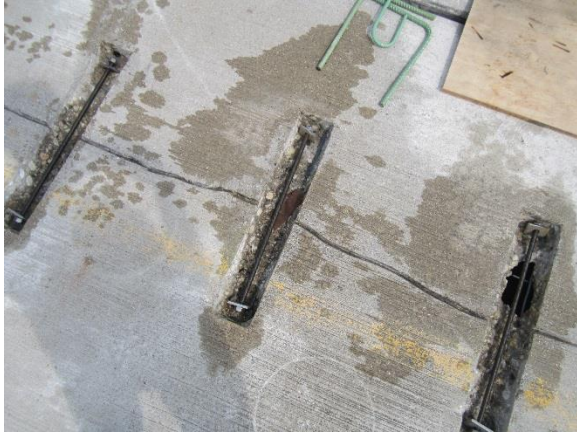
Figure 23. Stitch repair using stainless steel dowels
