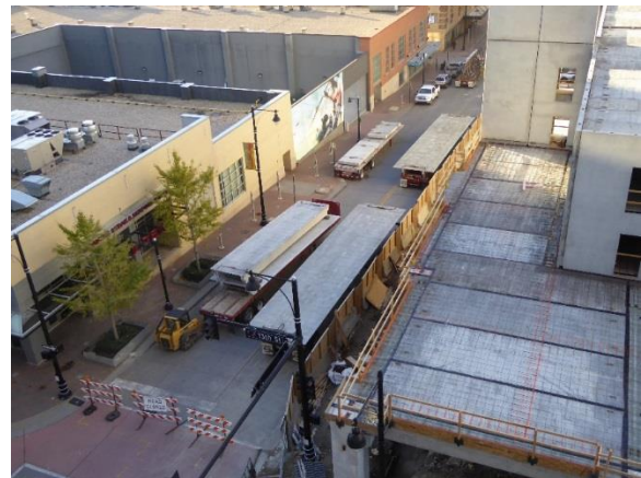
Figure 2. Precast double tee beams delivered to site prior to erection
