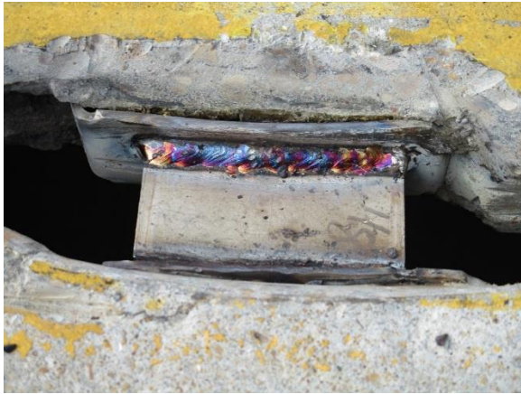
Figure 10. Rewelding slug to faceplate at flange-to-flange connection
