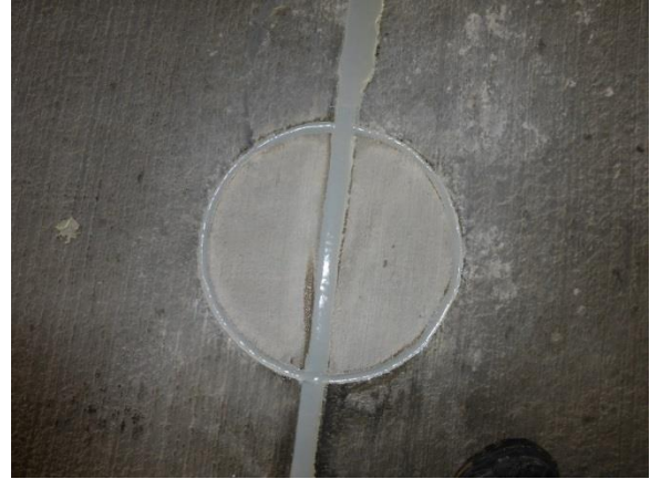
Figure 17. Completed core-hole repair
