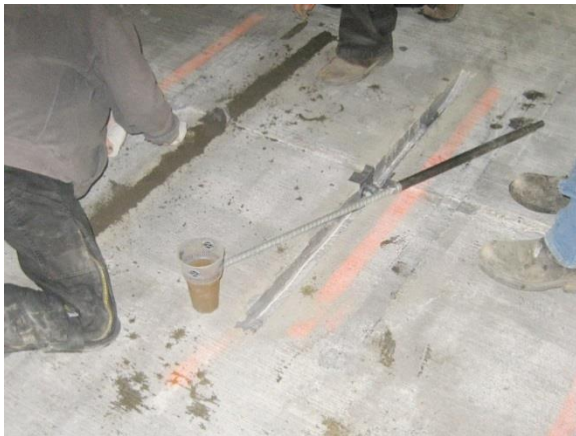
Figure 20. Embedded dowel repair using reinforcing bars
