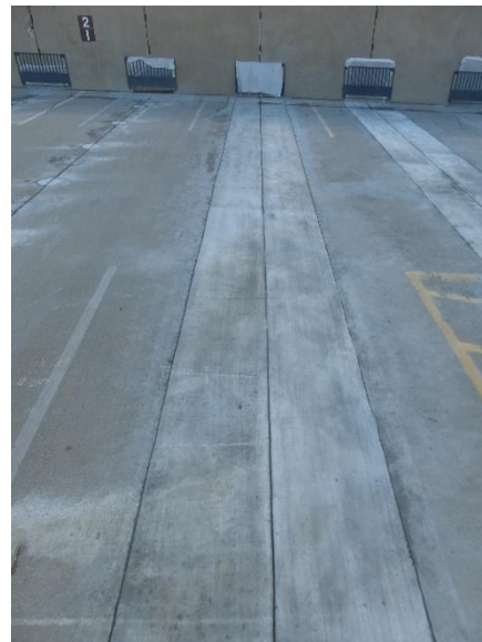
Figure 26. Completed full-depth flange repair
