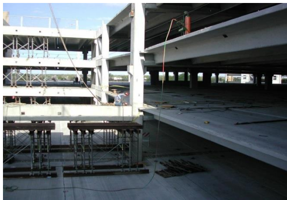
Figure 1. Precast parking structure during erection
