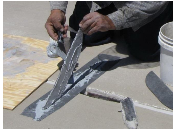
Figure 21. FRP composite biscuit installation
