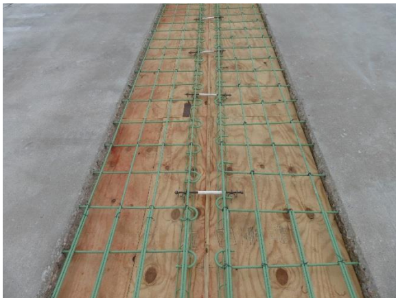
Figure 25. Full-depth flange repair in progress
