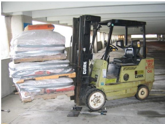
Figure 18. Load test on core-hole repair
