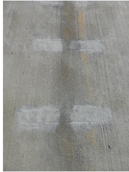
Figure 24. Completed stitch repair
