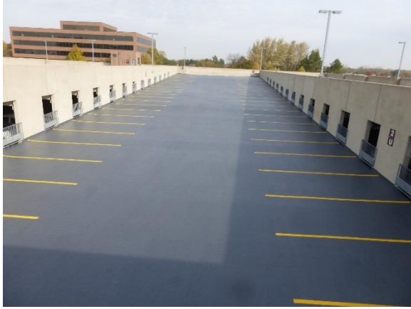
Figure 29. Vehicular traffic membrane on roof level ramp
