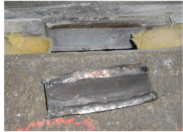
Figure 5 Fatigue failure of flat bar-type connection.
