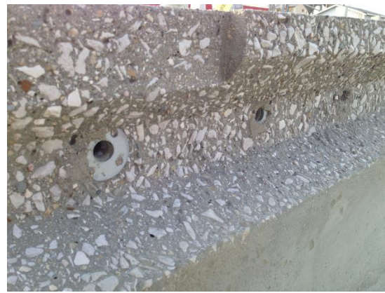
Fig. 6 Power washed shear key
