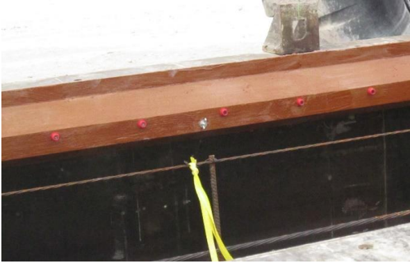
Fig. 3 Shear key form
