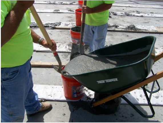
Fig. 8 UHPC placement
