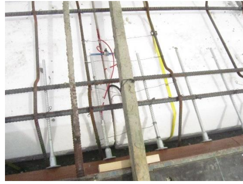
Fig. 4 Beam dowel parts in place
