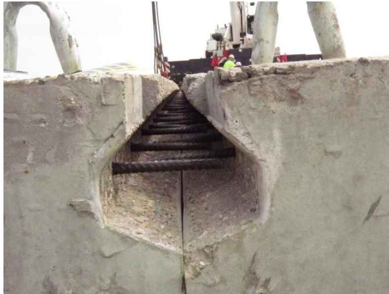
Fig. 7 Shear key with dowels
