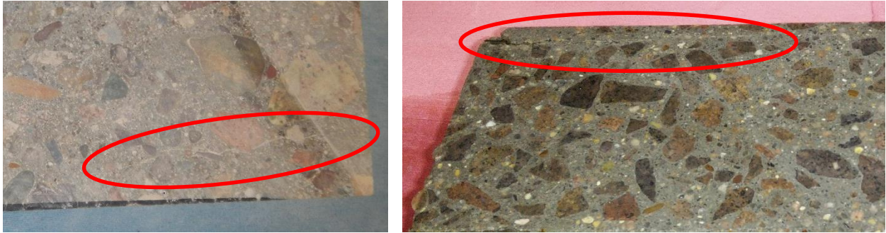
Figure 11: Cracking due to the stress release from saw-cutting
