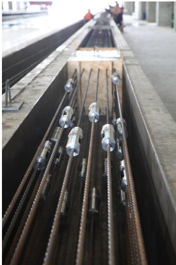
Fig. 5. Staggered couplers after initial pretensioning
