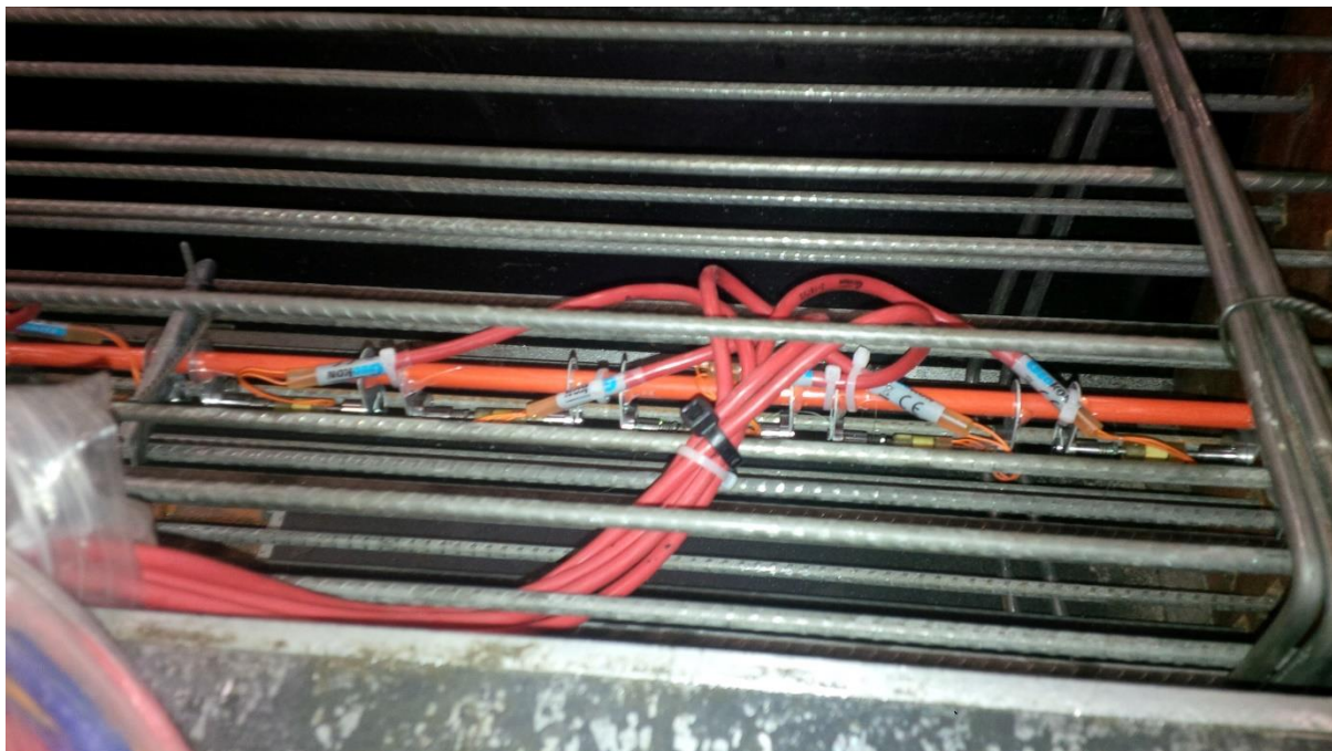
Figure 5: VWSGs secured in concrete tie form prior to casting concrete
