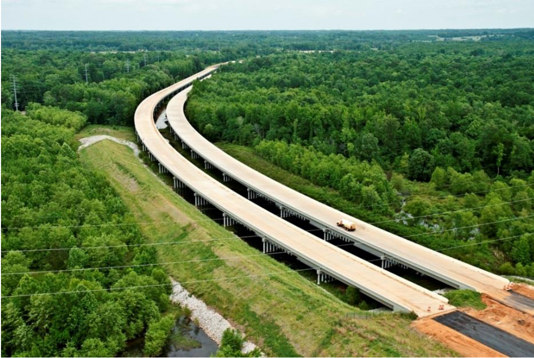
Figure 2. Completed Dual Structures
