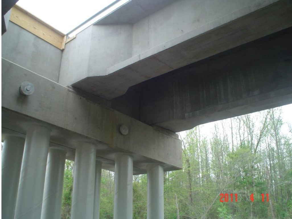
Figure 9. Installed Pipe Restrainers
