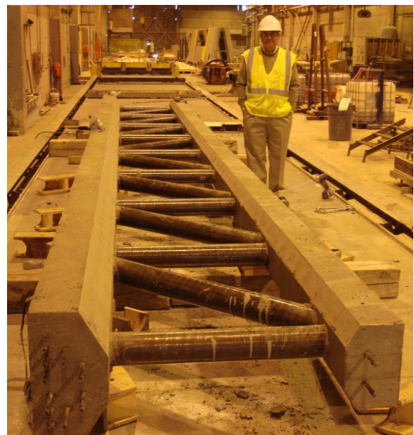
Fig. 8 The 8-panel girder after casting
