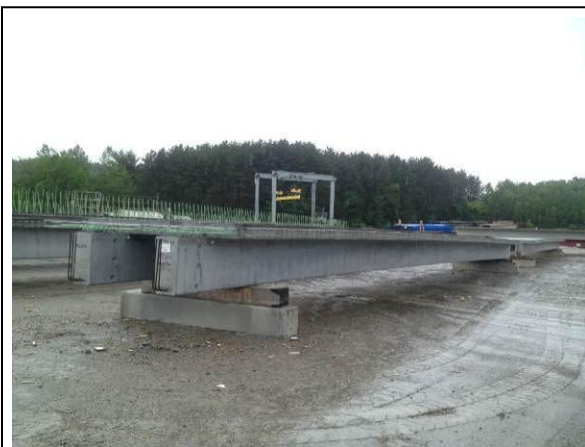
Figure 3: NEXT Beam in Fabrication Yard (Photo Courtesy of NYSDOT)
