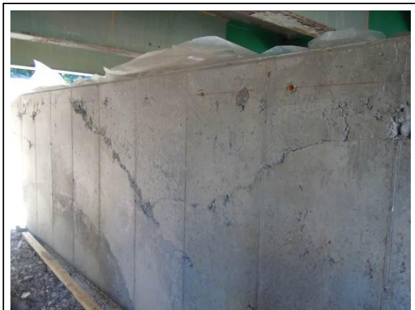
Figure 9: Eastbound East Abutment
