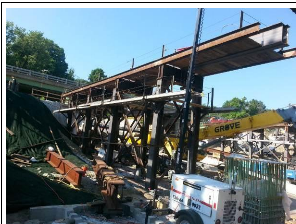
Figure 11: Primary Bent (Photo Courtesy of NYSDOT)
