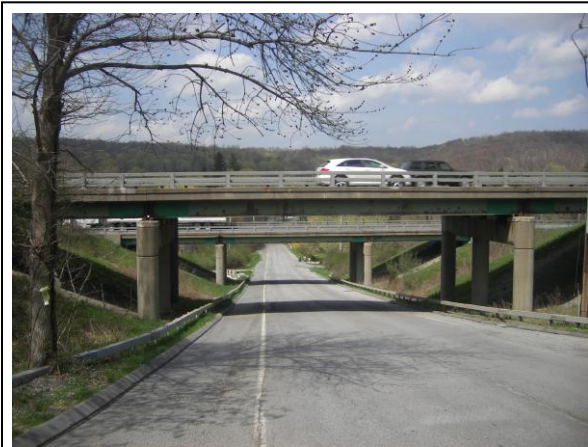
Figure 1: Original I-84 Bridges over Dingle Ridge Road
