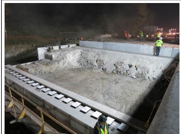
Figure 18: Temporary Slide Bearings on Abutment
