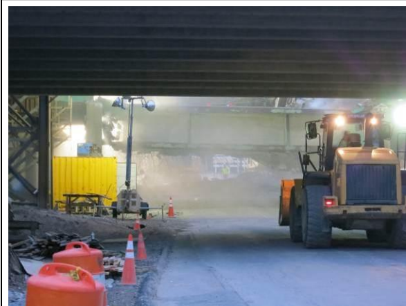
Figure 15: Demolition of Span 2
