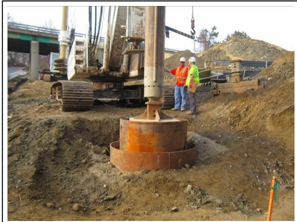
Figure 8: Drilled Shaft Core Barrel
