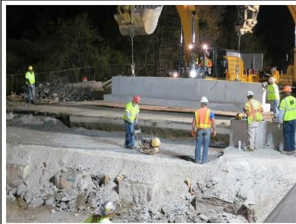
Figure 19: Sleeper Slab Placement
