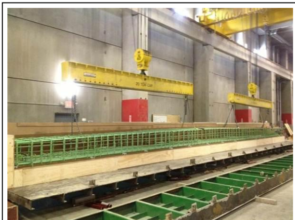
Figure 5: End Diaphragm Fabrication (Photo Courtesy of NYSDOT)
