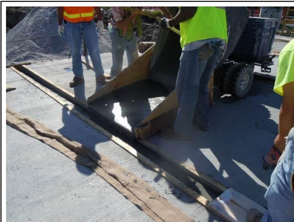
Figure 13: Placing of UHPC
