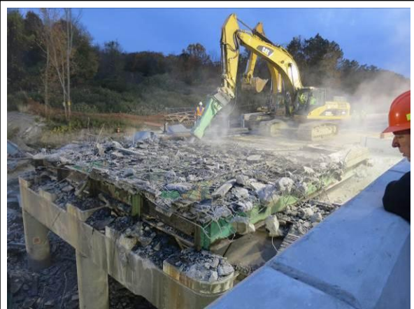
Figure 16: Demolition of Approach Span
