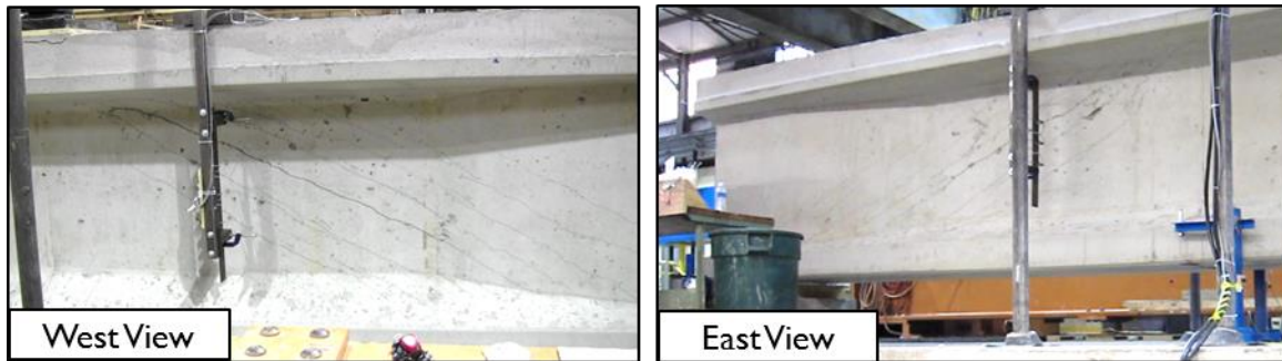
Tx62-3 (South): immediately prior to shear failure
