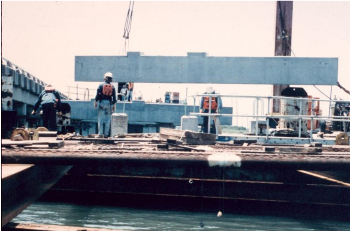
Fig. 5: Crane placement of precast bent cap
