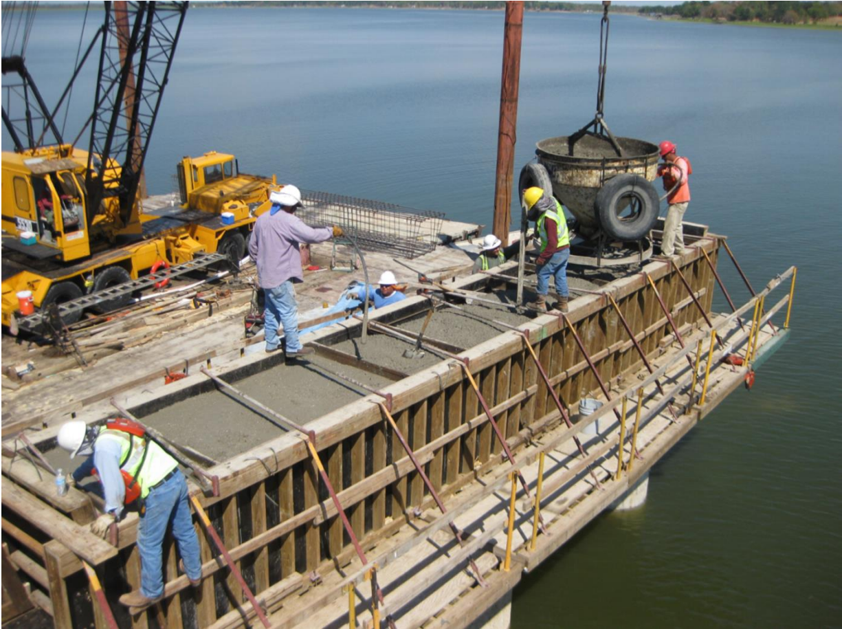
Fig. 2: Cast-in-place concrete placement
