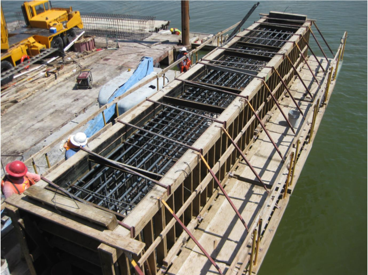
Fig. 1: Formwork for cast-in-place bent cap
