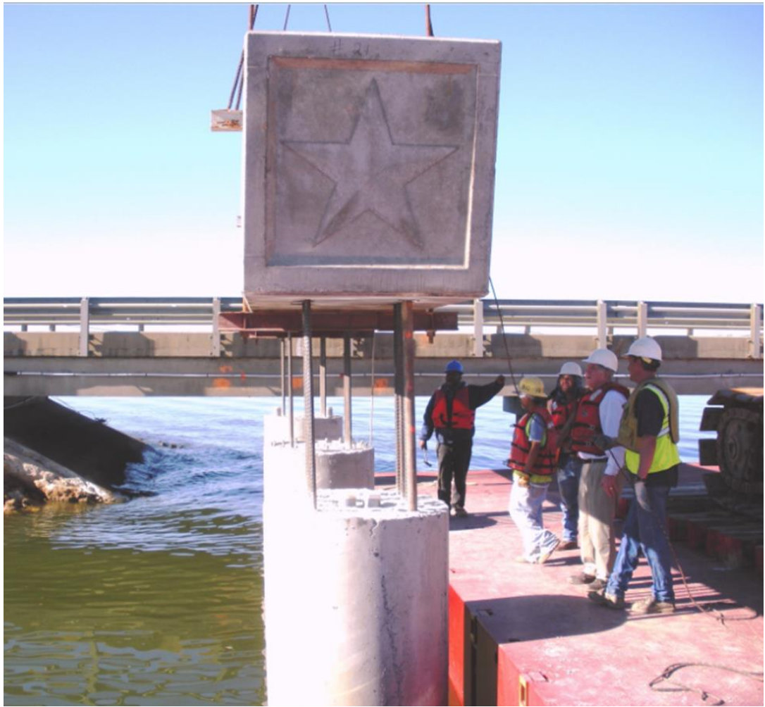
Fig. 9: Cap to column connection
