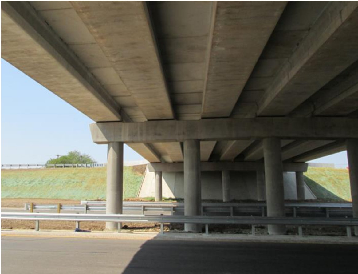
Fig. 3: Substructure adjacent to underlying roadway
