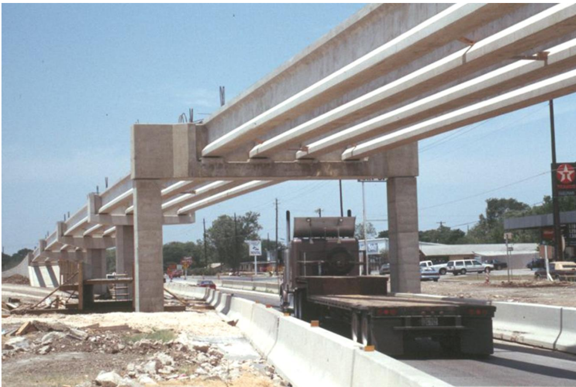
Fig. 4: US 290 Ramp G Straddle Bent
