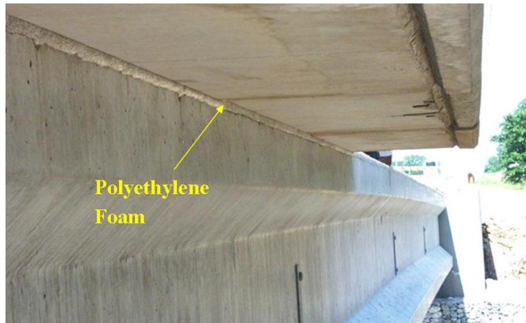
Figure 3. Beam/Overhang Panel Interface
