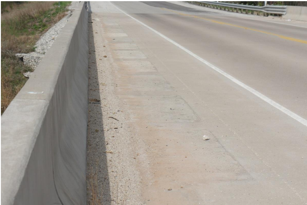
Figure 8. Current Picture of Rock Creek Bridge Deck, FM 1885
