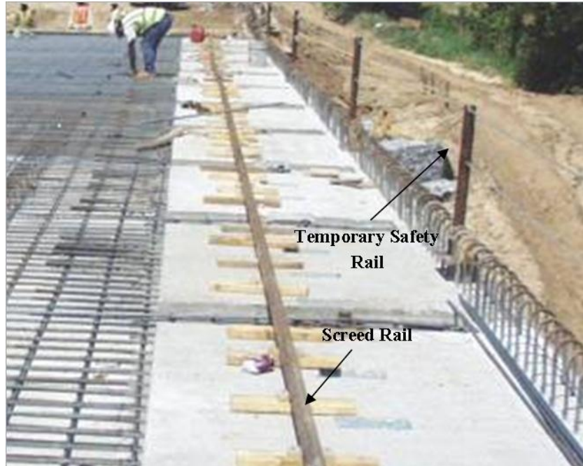
Figure 4. Overhang Panels after Placement
