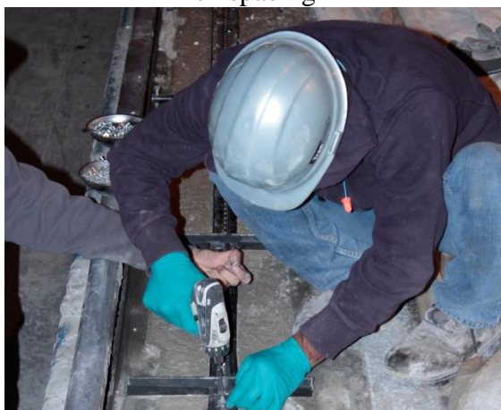
(c) Removal of steel bar from hardened concrete
