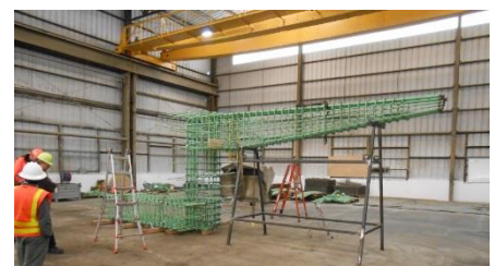
Mock-up Fabrication of Precast Zee Segment Rebar Cage (photo by author).
