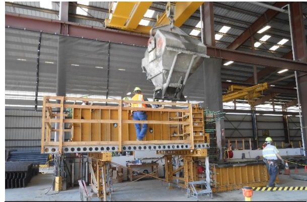
Formwork and SCC Placement for Precast Mock-Up Segment (photo by author).
