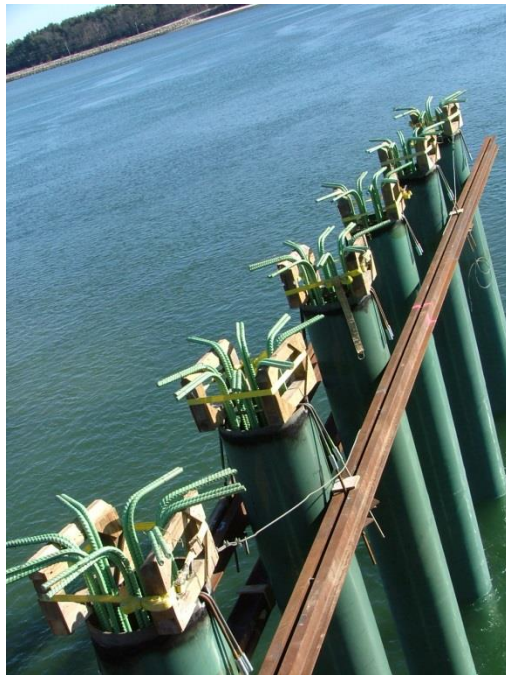
Figure 9: Pipe Pile Reinforcing (2 of 2)
