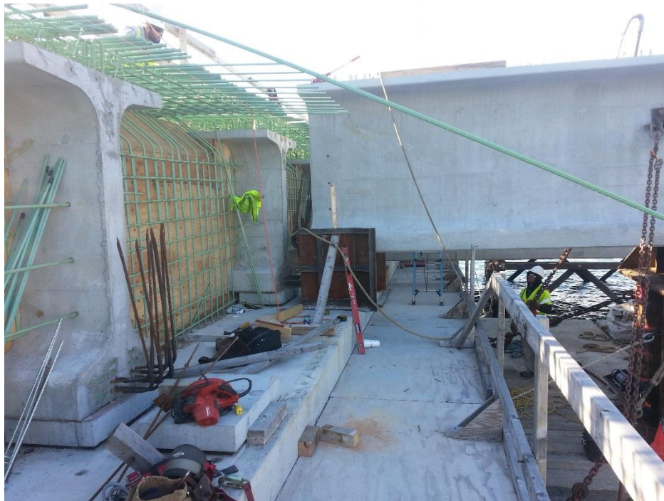
Figure 7: Steel pocket guiding beam into place at Pier 9.
