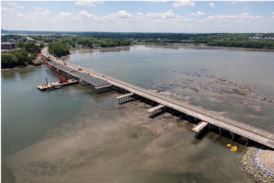
Figure 1: Aerial view of the Martin's Point Bridge under construction
