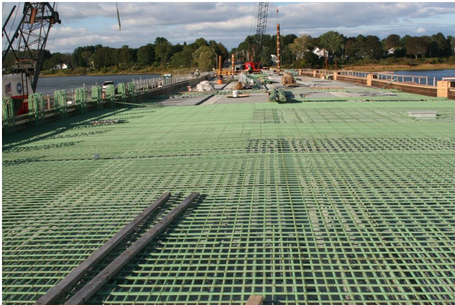
Figure 10: Typical deck reinforcing layout.
