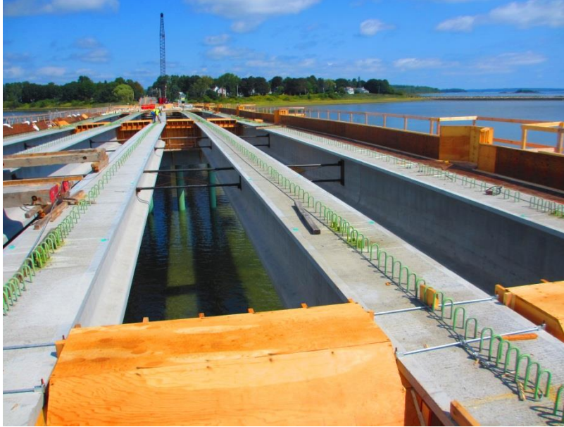
Figure 4: Temporary Intermediate Pipe Cross Frames.
