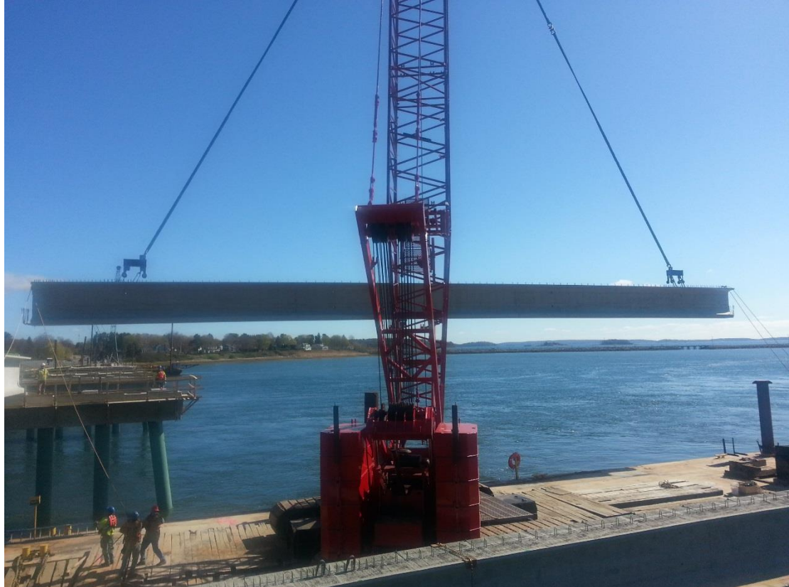
Figure 5: Beam erection from barge.
