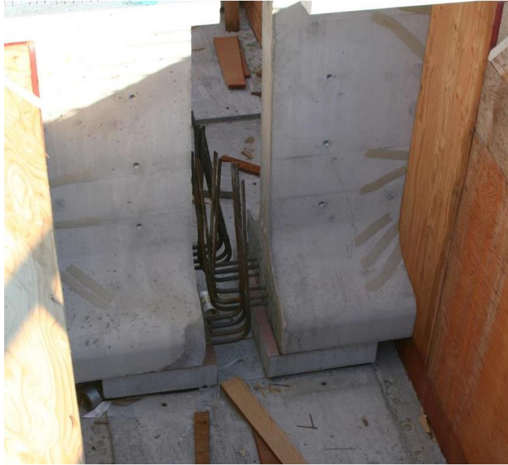
Figure 3: Strand Projections at Beam Ends.
