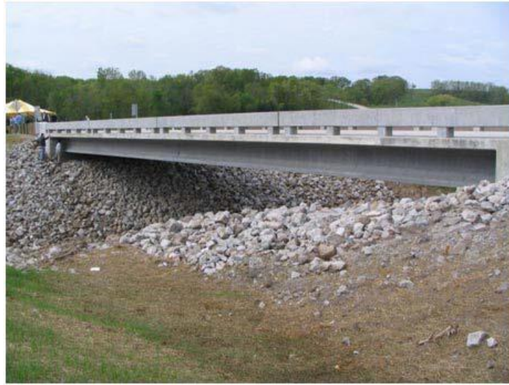
Fig. 7 The First UHPC Prestressed I-girder Bridge in US 6
