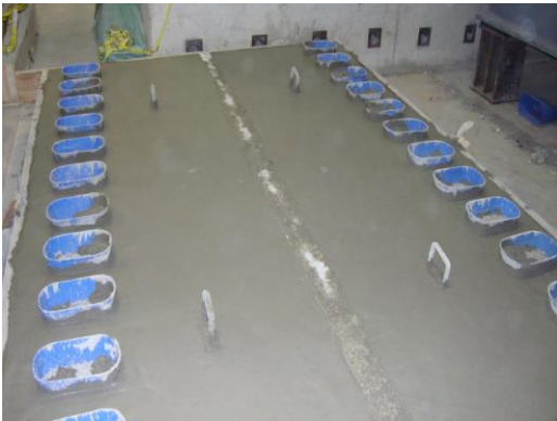
c) Casting the slab
