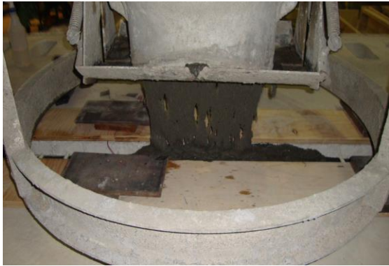
g) Close-up view of dropping UHPC into the joint
