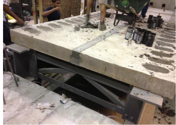
b) Filling shear pockets with grout
