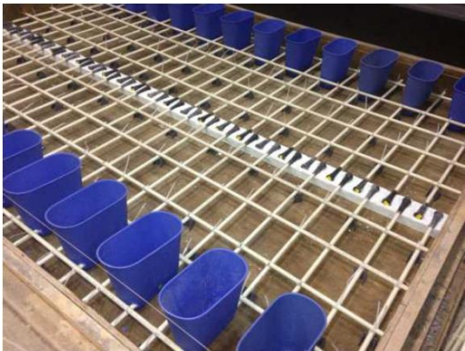
a) Lower layer of GFRP bar at joint
