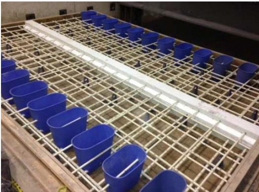
b) GFRP bars and styrofoam forming the joint
