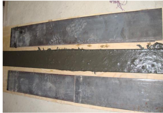
h) After Filling closure strip with UHPC
