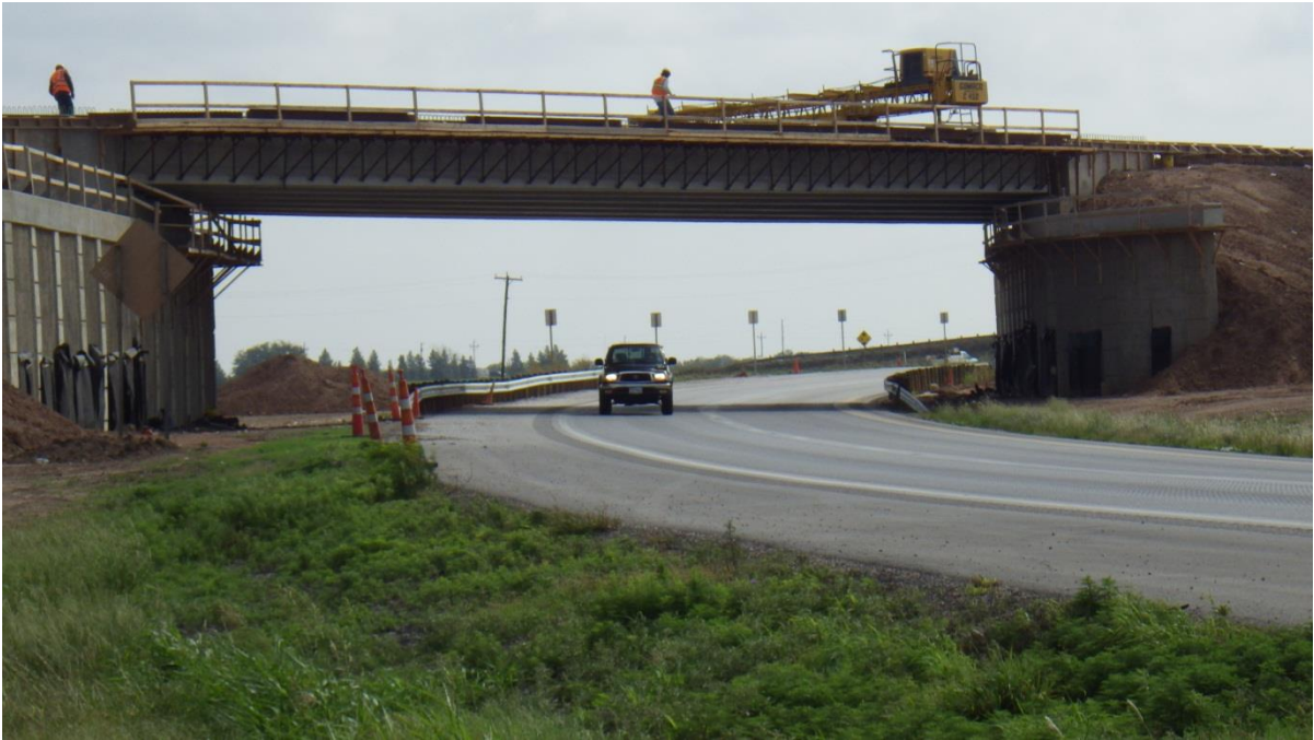
Figure 2 New single span bridge structure under construction
