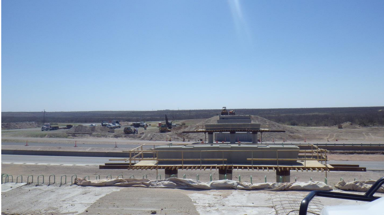
Figure 17 New Bridge with Four Spans
