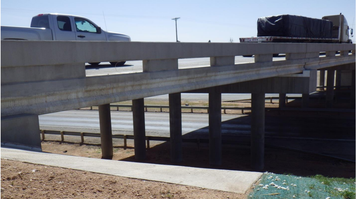
Figure 11 Completed Bridge Structure with T 223 Rail (Vertical Clearance 18.0')
