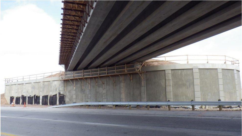
Figure 3 New Retaining wall wraps around the abutment
