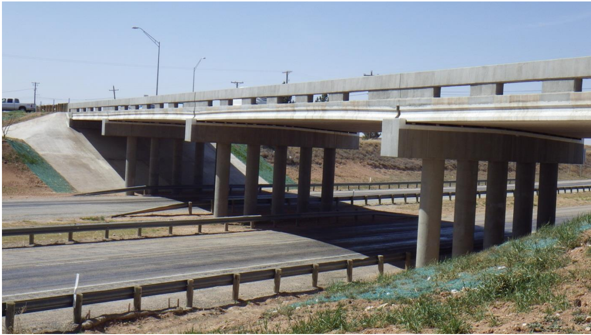
Figure 10 Completed Bridge Structure – US 184 Underpass at US 84 in Snyder County.
