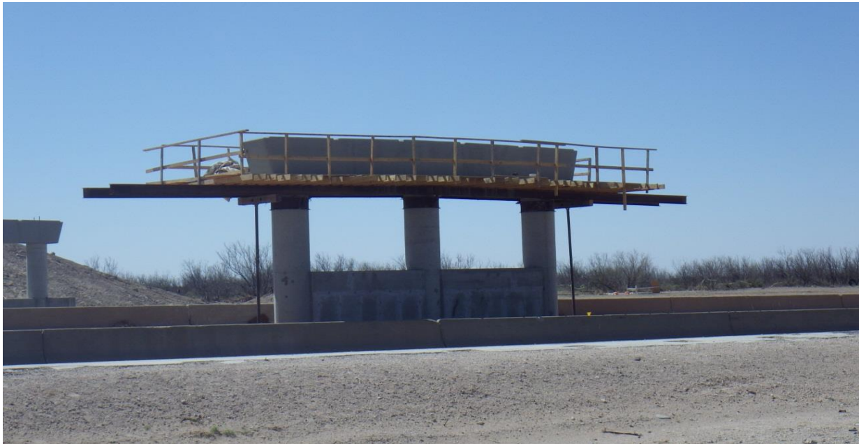
Figure 16 New Bridge Under Construction- IH 20 Underpass at FM 2599 in Howard County
