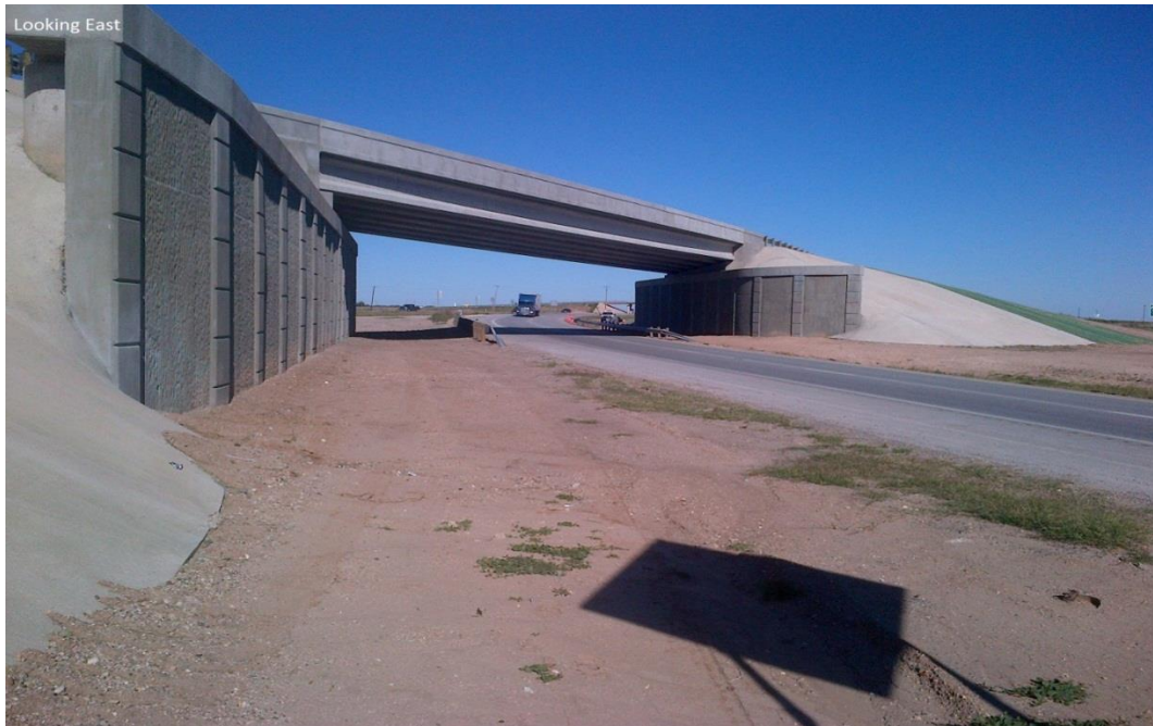
Figure 4 Completed Bridge Structure –WB IH 20 Underpass at EB US 83
