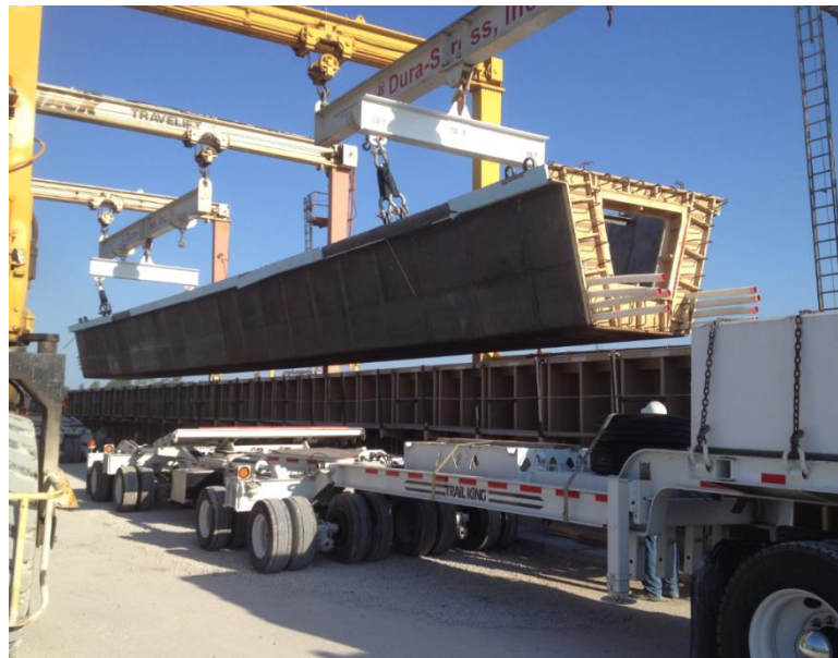
Figure 14: Girder Segment Lift
