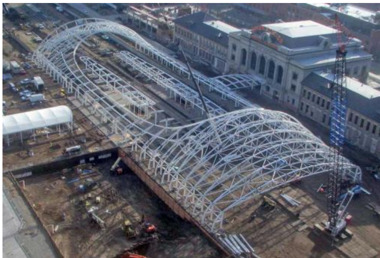
Figure 11: Final Stage construction near completion, with fully erected CRT canopies.
