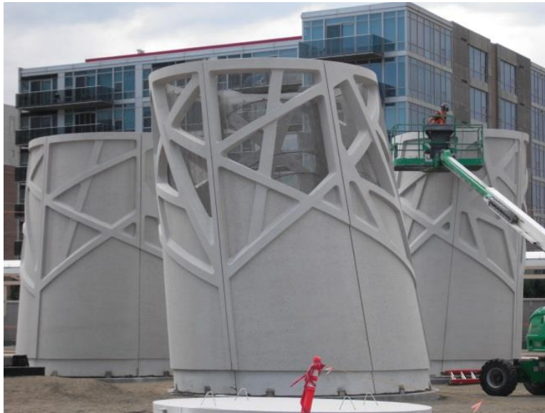
Figure 30: Precast Vent Tower during Erection
