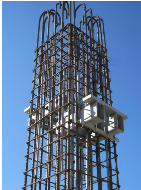
Figure 13: Cast-in-place column with steel corbels.
