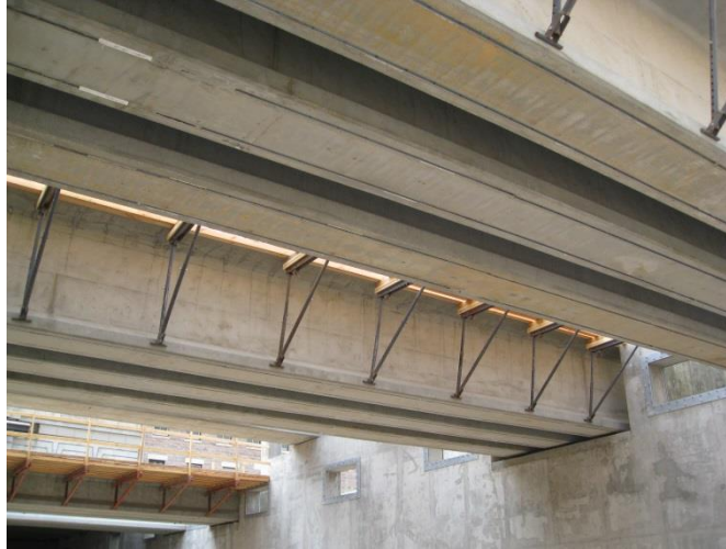
Figure 27: AMTRAK train bridges with full BT girder, CRT bridge can be seen beyond.
