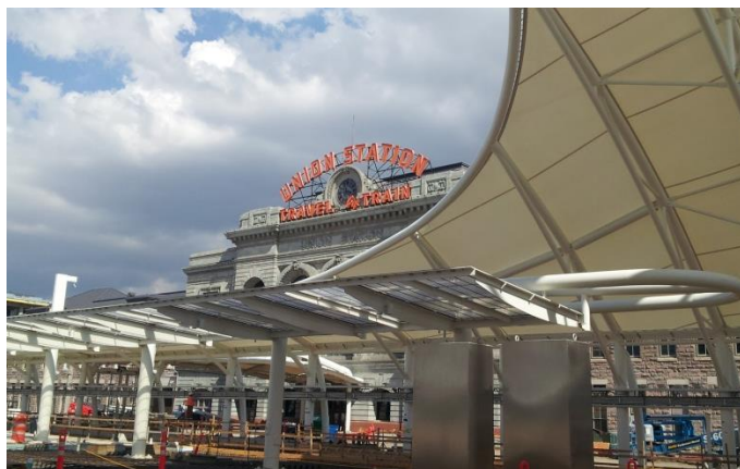
Figure 3: Train Hall Canopies during platform construction.
