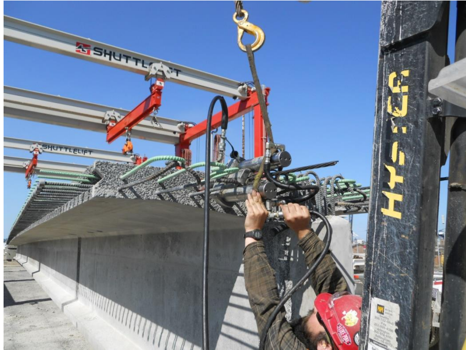
Figure 6: Installation of Temporary Post-Tensioning Strands in Girder Top Flange
