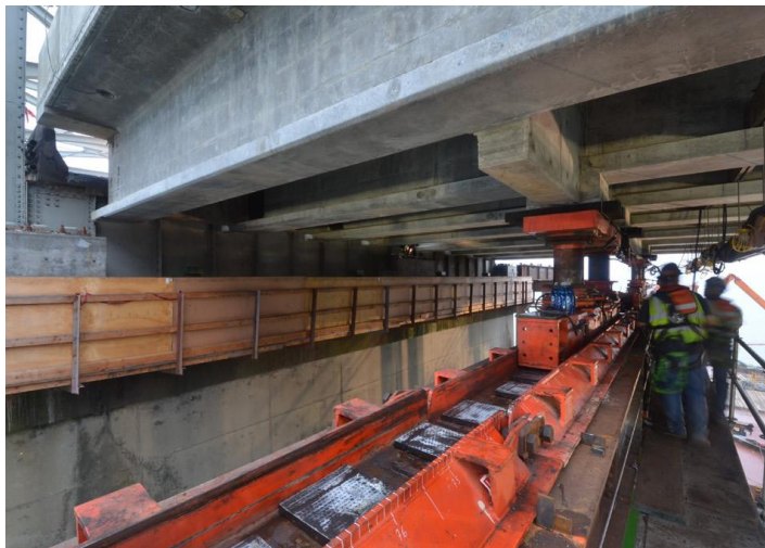
Figure 4: View from Underneath Permanent Replacement Span during lateral slide-in.
