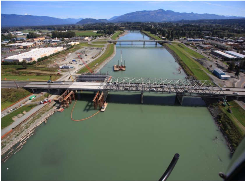
Figure 5: Completed Bridge Open to Traffic Immediately Following Span Switchover
