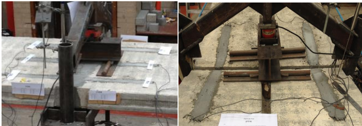
(a) Concrete at the joint gaps FT1, FT2, FT3
