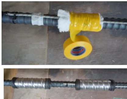
(a) Rebar preparation
