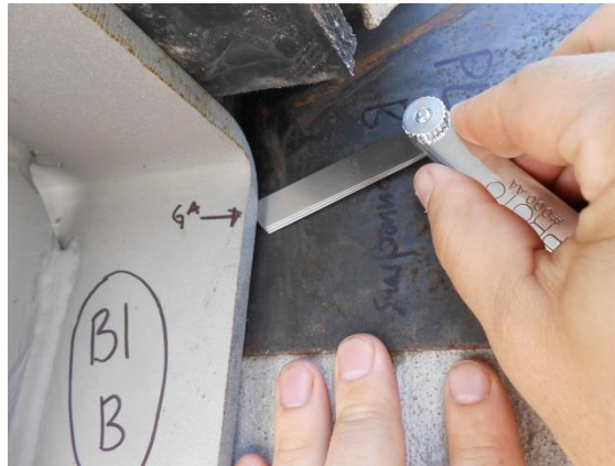
Figure 7 - Measuring gap behind gusset plate
