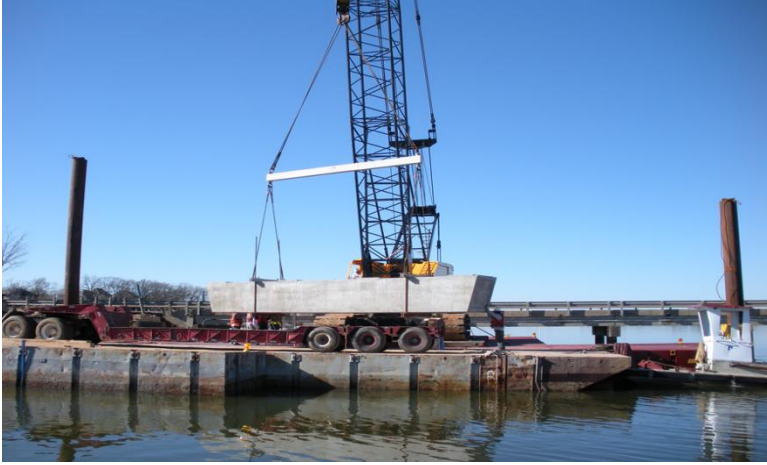
Figure 15. Two point lifting of precast bent cap
