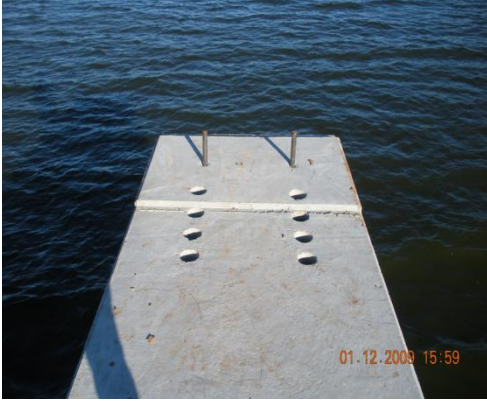
Figure 8. Precast Cap and Connection Detail
