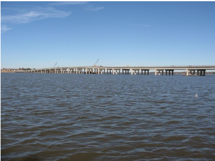
Figure 5. Twin Creek Bridge
