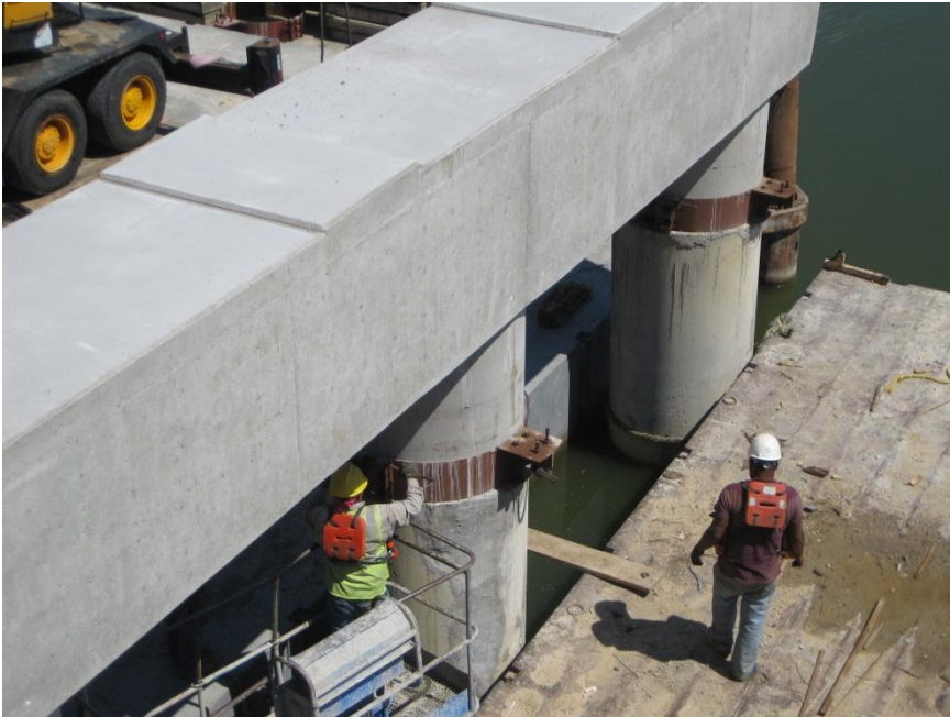
Figure 21. Column with friction collars
