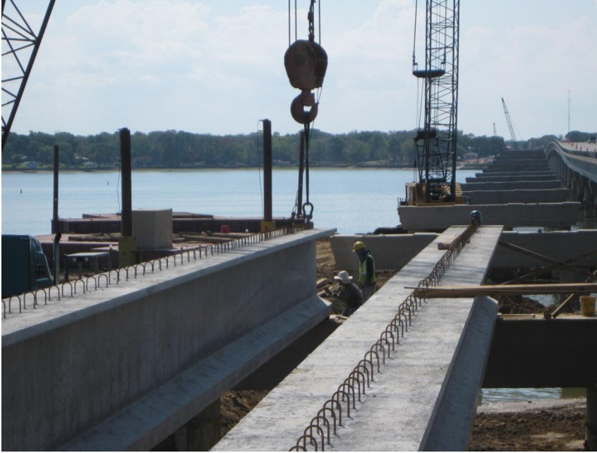
Figure 20. TX 70 Girder - Lifting and Placement
