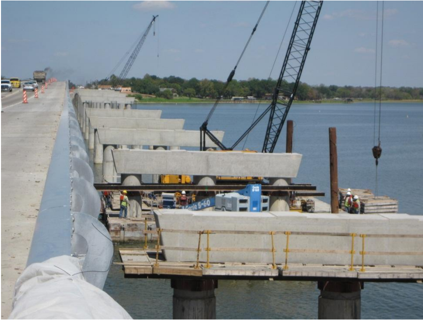
Figure 18. Placement of precast bent cap for 21 bents at Caney Creek
