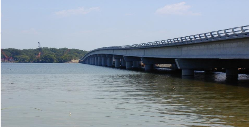
Figure 14. Caney Creek Bridge (completed structure)
