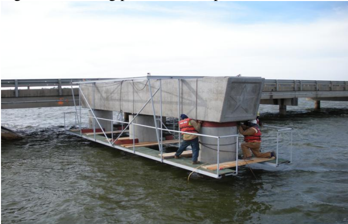
Figure 17. Lowering Precast Bent Cap into friction collars
