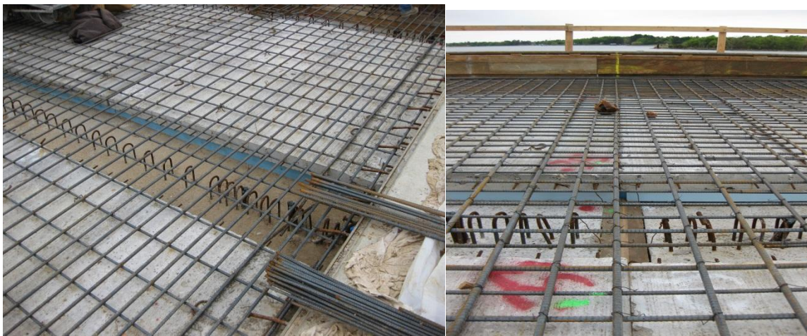
Figure 12. Precast Panel Placement
