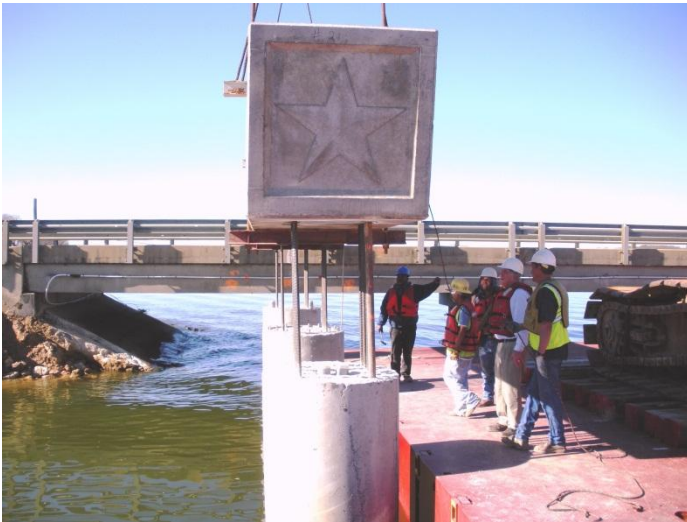
Figure 16. Placing precast bent cap into column connection dowels in phase 1
