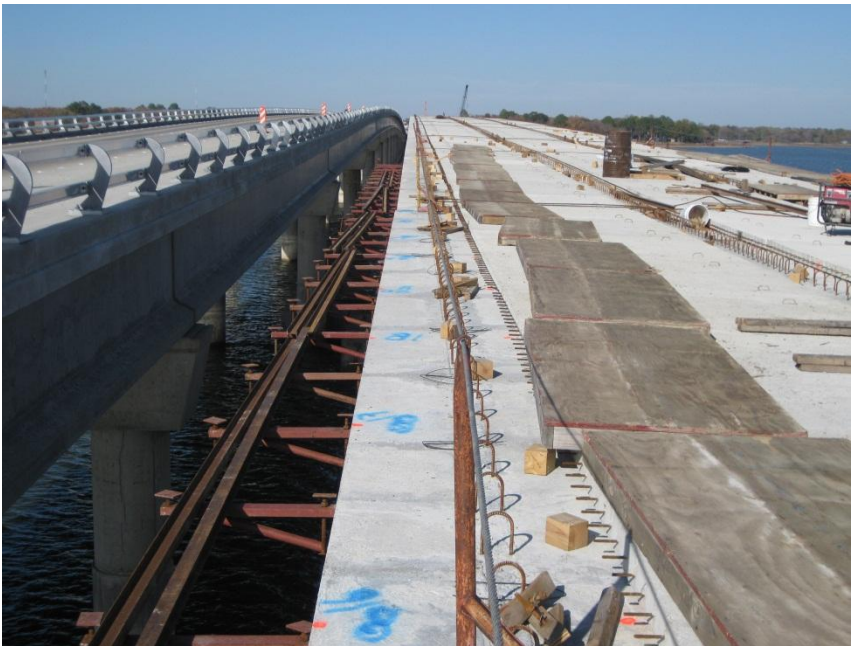
Figure 19. Caney Creek – Phase 2 (Phase 1 completed and open to traffic)
