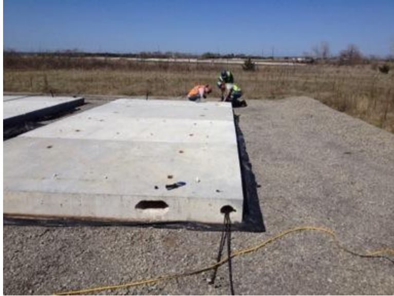
Figure 10 Strands being threaded manually through the ducts
