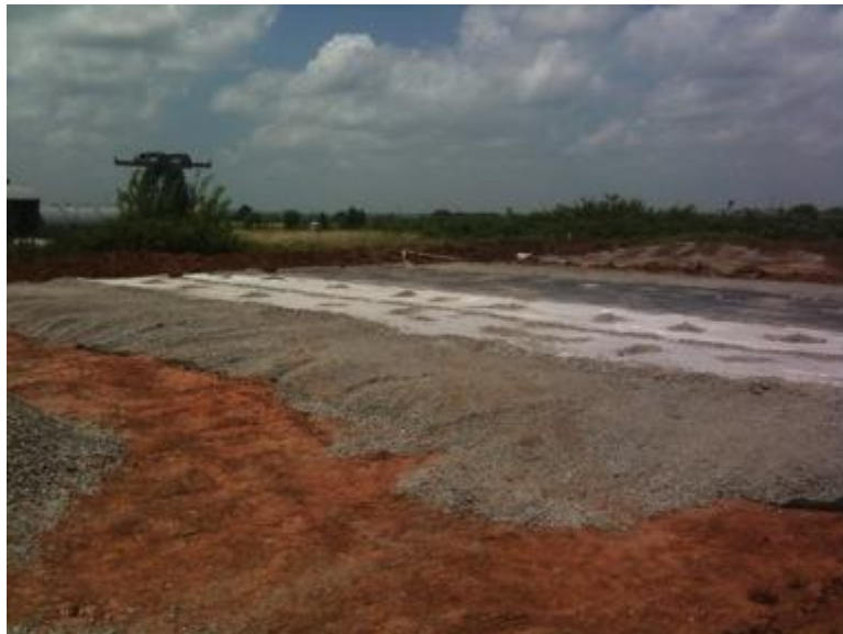
Figure 7 Subgrade construction and compaction of base materials
