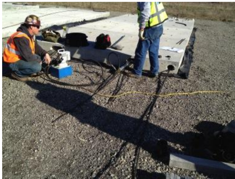
Figure 11 Tendons stressing for Pavement III
