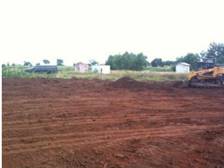
Figure 6 Project site subgrade preparation
