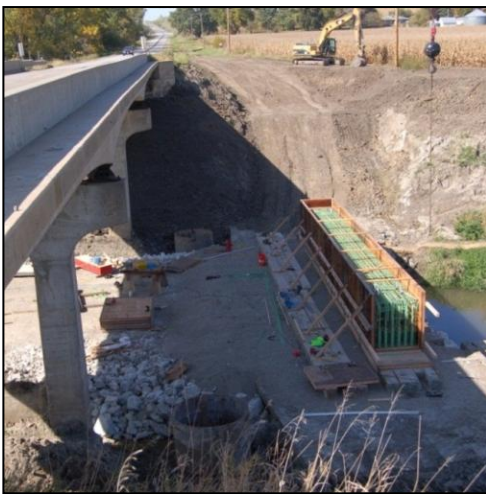
Figure 12. Pier cap beam casting adjacent to bridge
