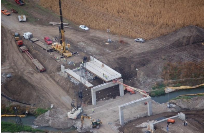
Figure 17. Erection of superstructure modules
