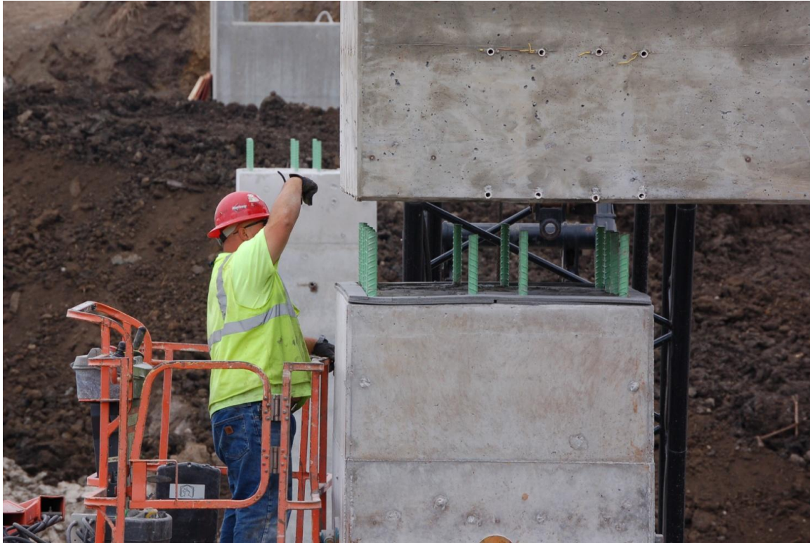
Figure 16. Connection of precast cap to precast column
