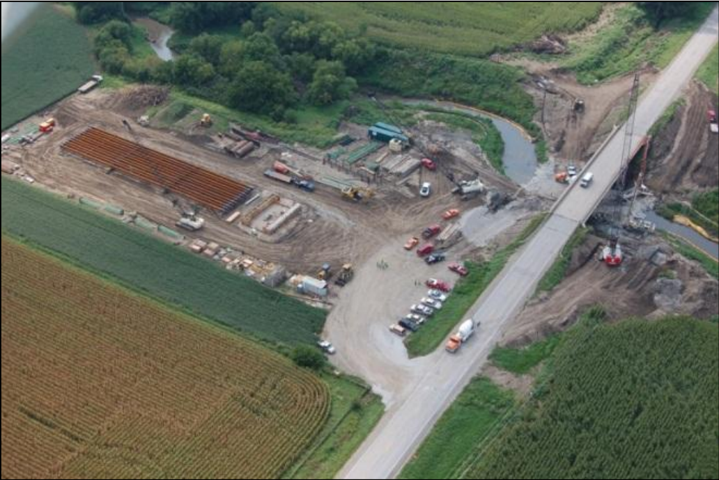
Figure 8. Aerial view of bridge site
