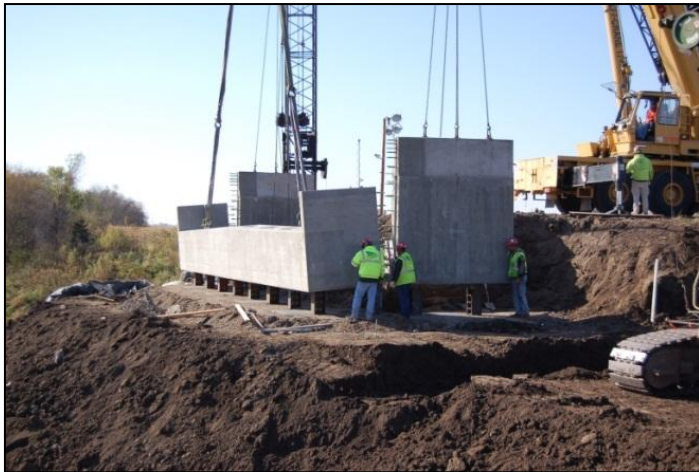
Figure 13. Installation of abutment and wingwalls
