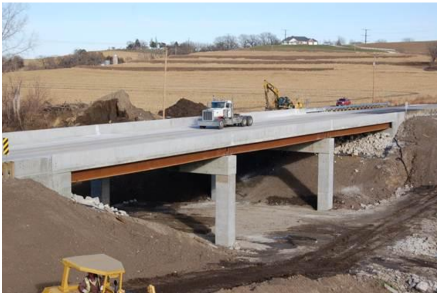
Figure 1. View of completed bridge. US Highway 6 over Keg Creek, Council Bluffs, Iowa.
