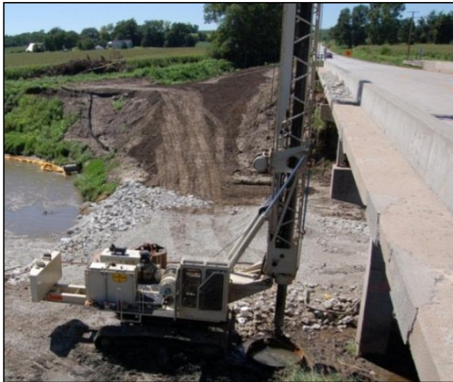
Figure 9. Drilled shaft construction
