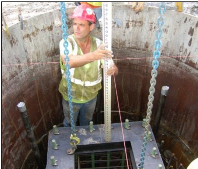
Figure 10. Installation of dowel bars for drilled shaft
