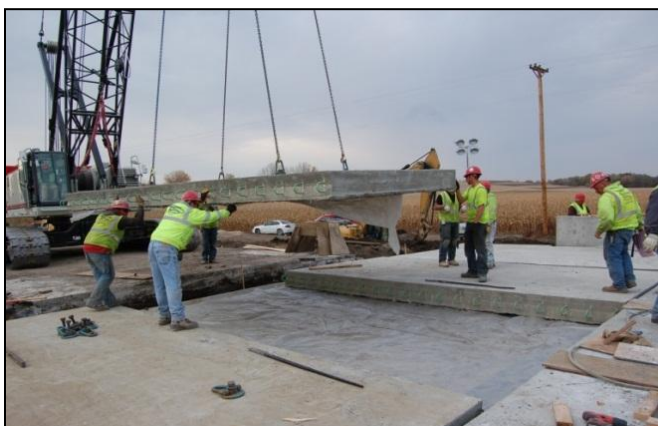
Figure 18. Installation of precast approach slabs
