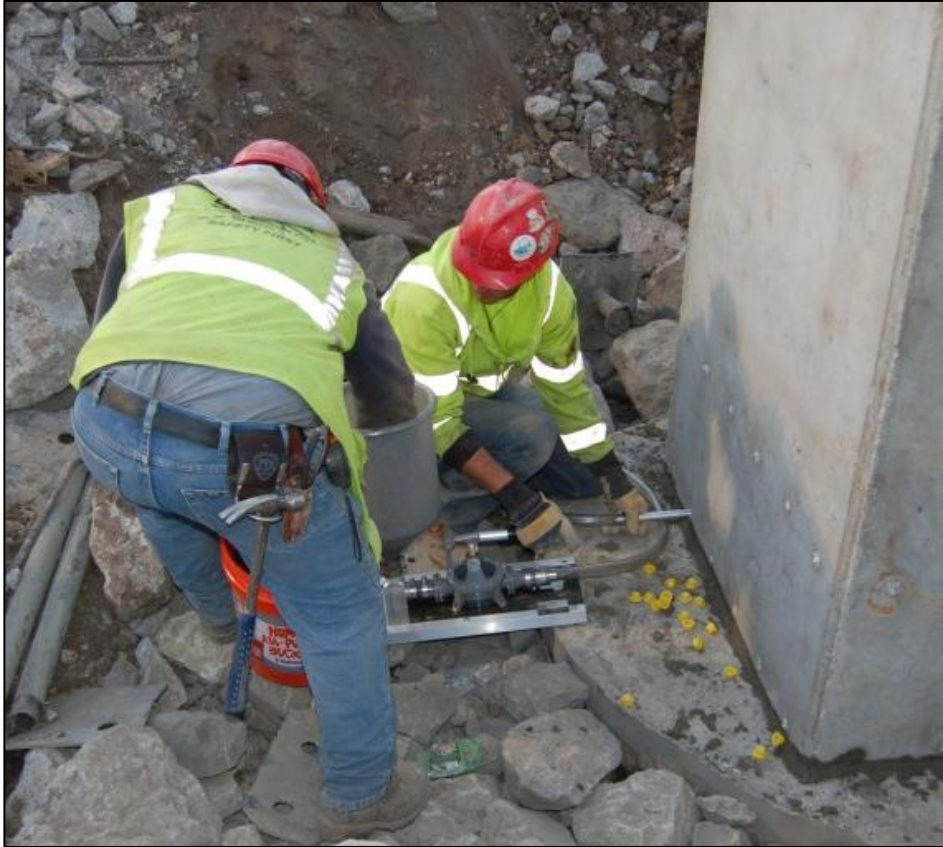
Figure 15. Injecting grout into couplers
