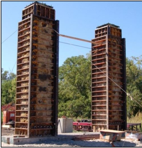
Figure 11. Pier columns formed in casting yard
