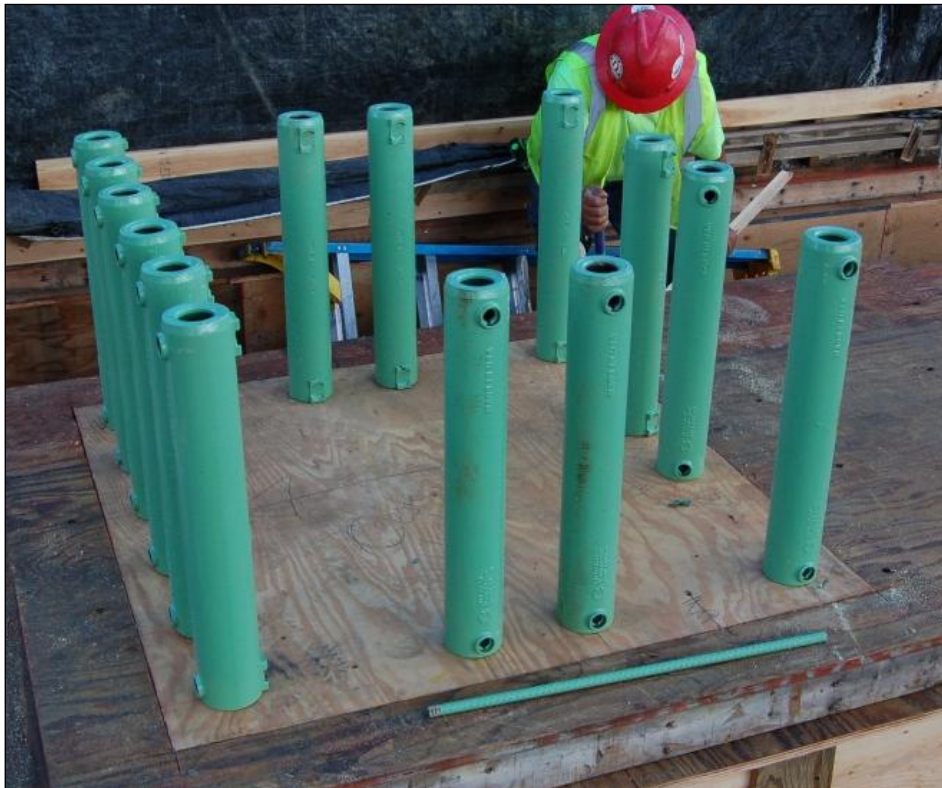
Figure 14. Rebar couplers
