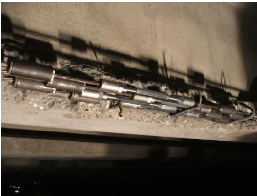
Figure 4 Repair of severed strands with coupling device
