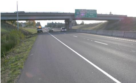
Figure 3 Lieser Road Bridge
