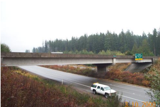
Figure 1 Trigger Avenue Bridge over State Route 3
