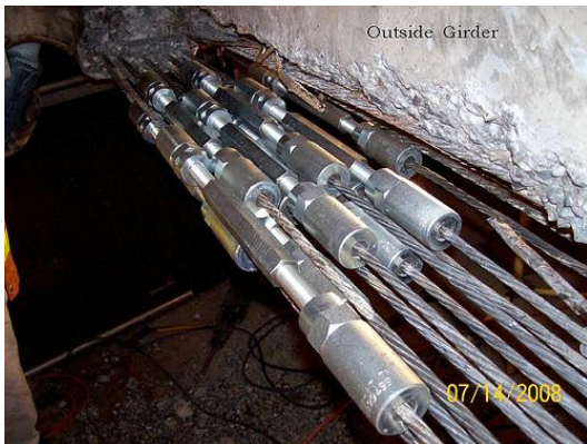
Figure 9 Temporary repairs using strand couplers
