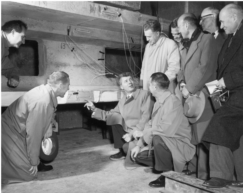
Fig. 1 Art Anderson, “Let’s Ask the Beam” —a test evaluating how an I-beam behaves with large openings for utilities in a high-rise office building.
