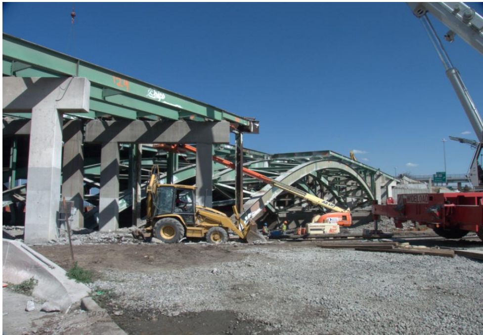
Fig. 12: Demolition of Existing Bridge
