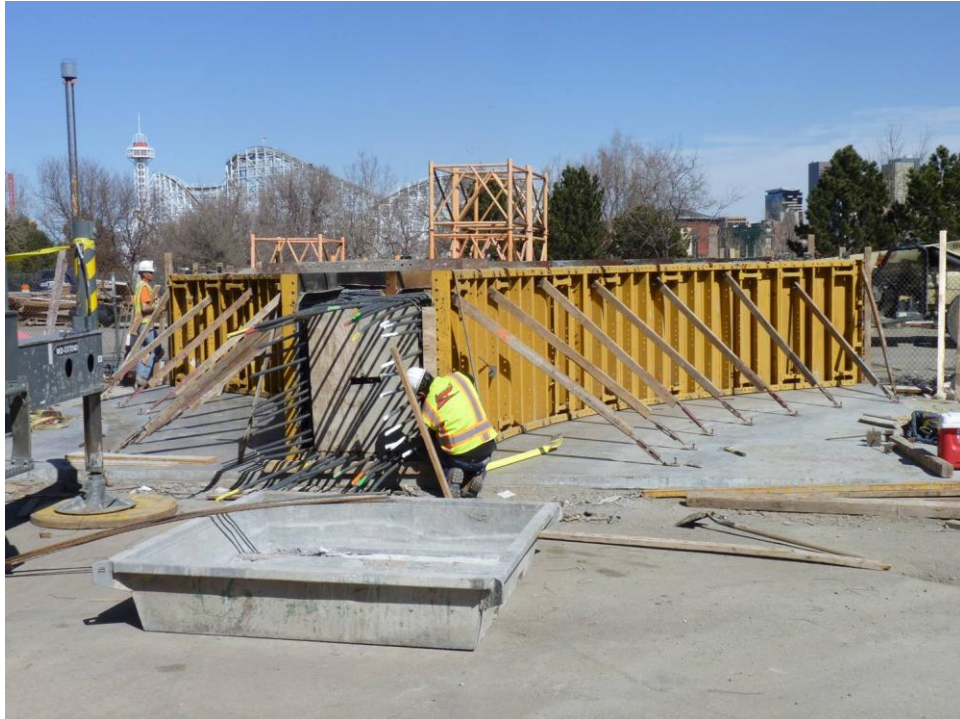
Fig. 10: Precasting of Interior Piers
