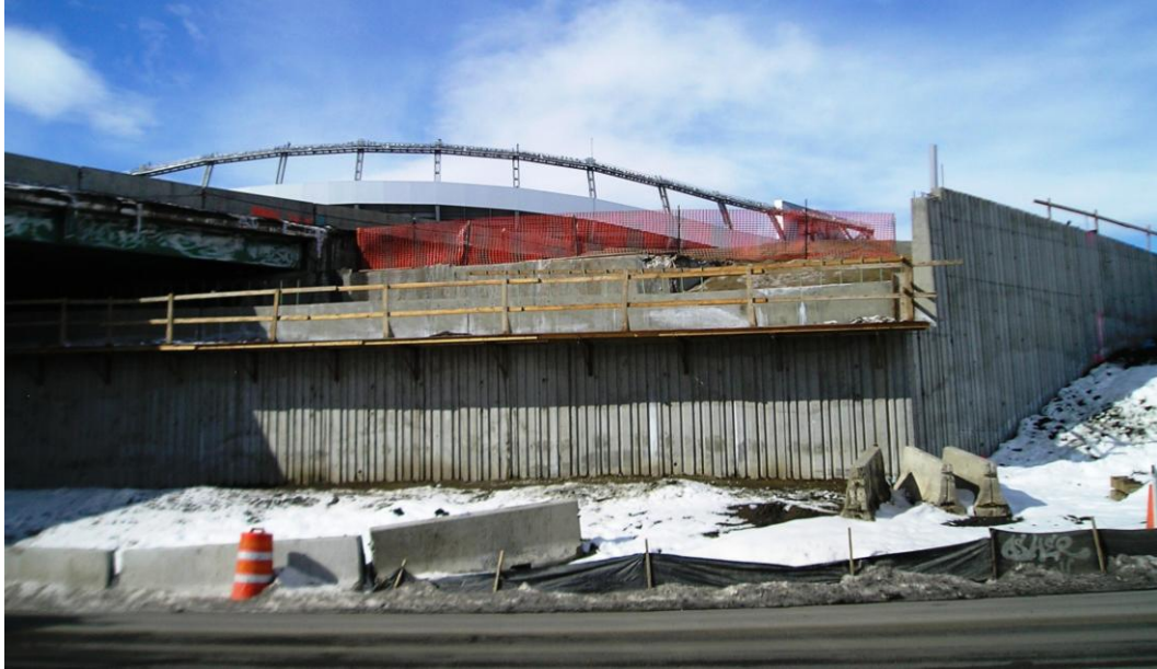
Fig. 8: Abutment and Wall Construction under existing Bridge
