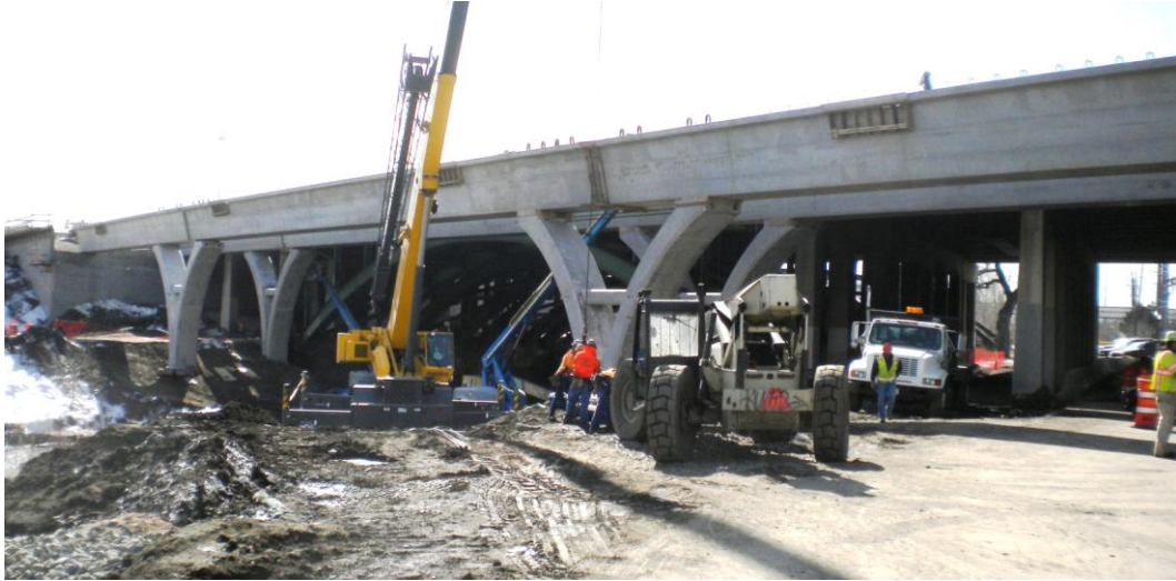
Fig. 17: Continuous Girder Line
