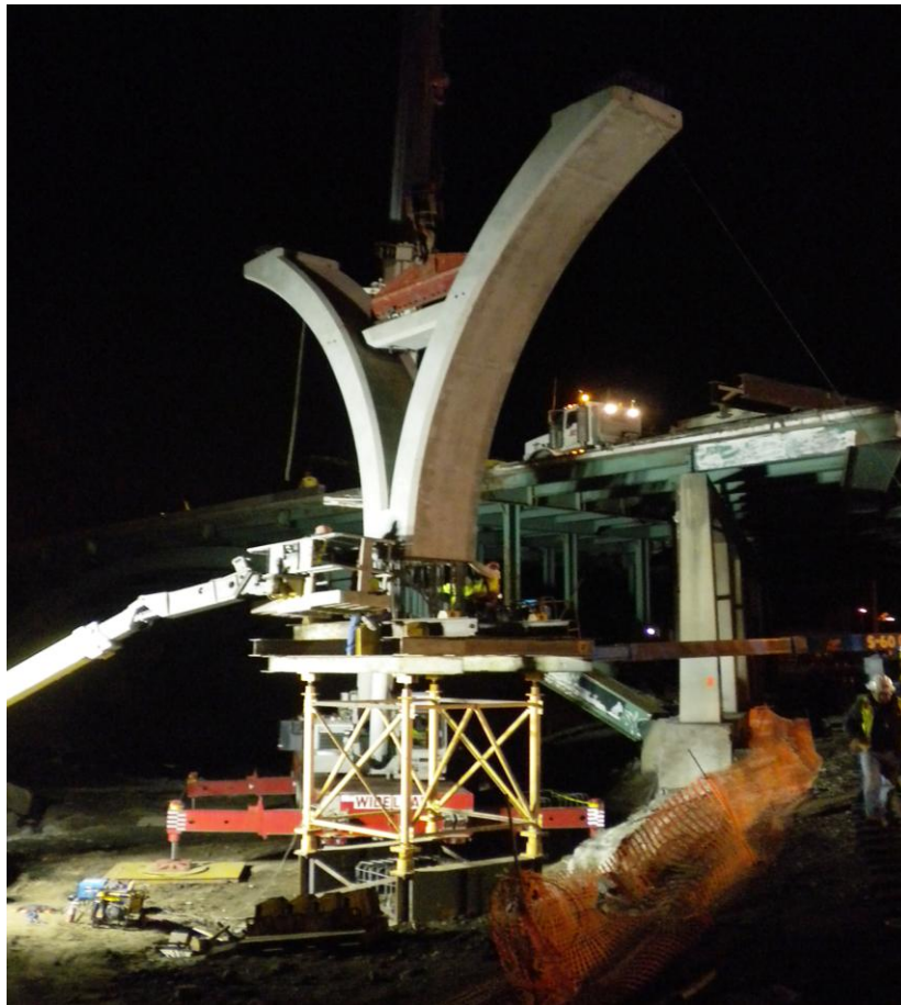
Fig. 13: Erection of Precast Piers
