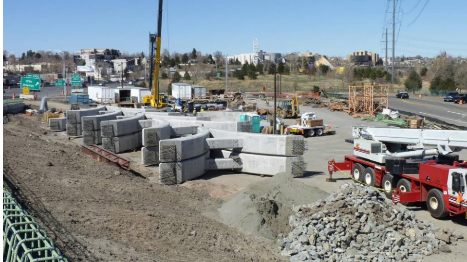
Fig. 11: Storage of Precast Interior Piers
