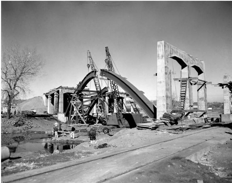
Fig. 1: Construction of original Bronco Arches, 1961
