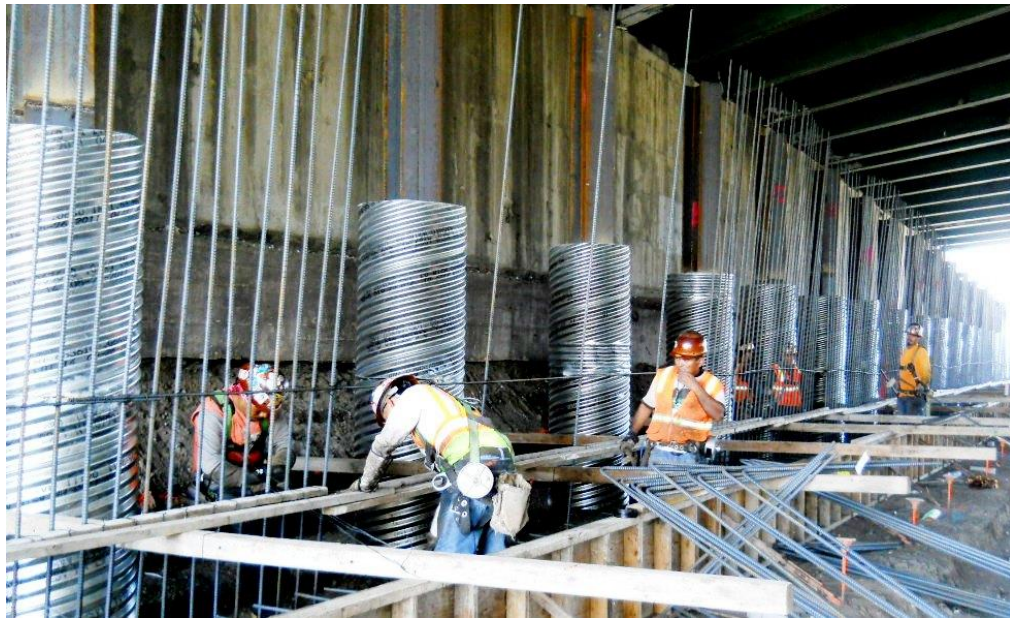
Fig. 7: Abutment Piling Encased in Corrugated Pipe through Retaining Wall Footing
