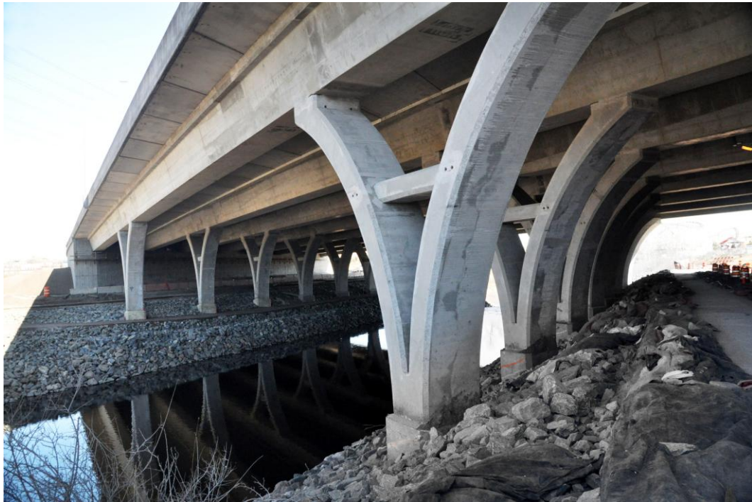
Fig. 19: Completed Bridge, March 2013
