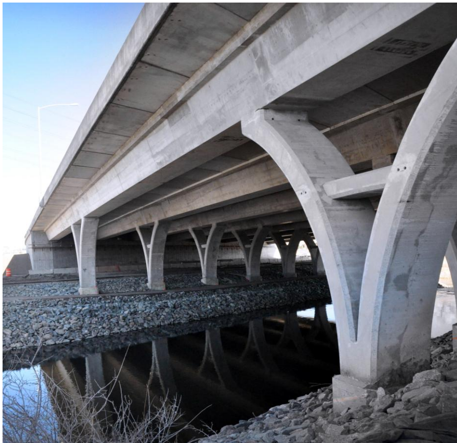
Fig. 9: Interior Pier and Pedestal Details
