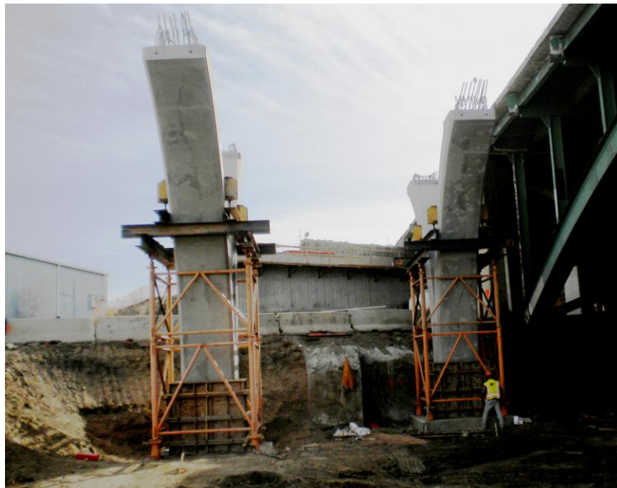
Fig. 14: Precast Piers on Temporary Shoring
