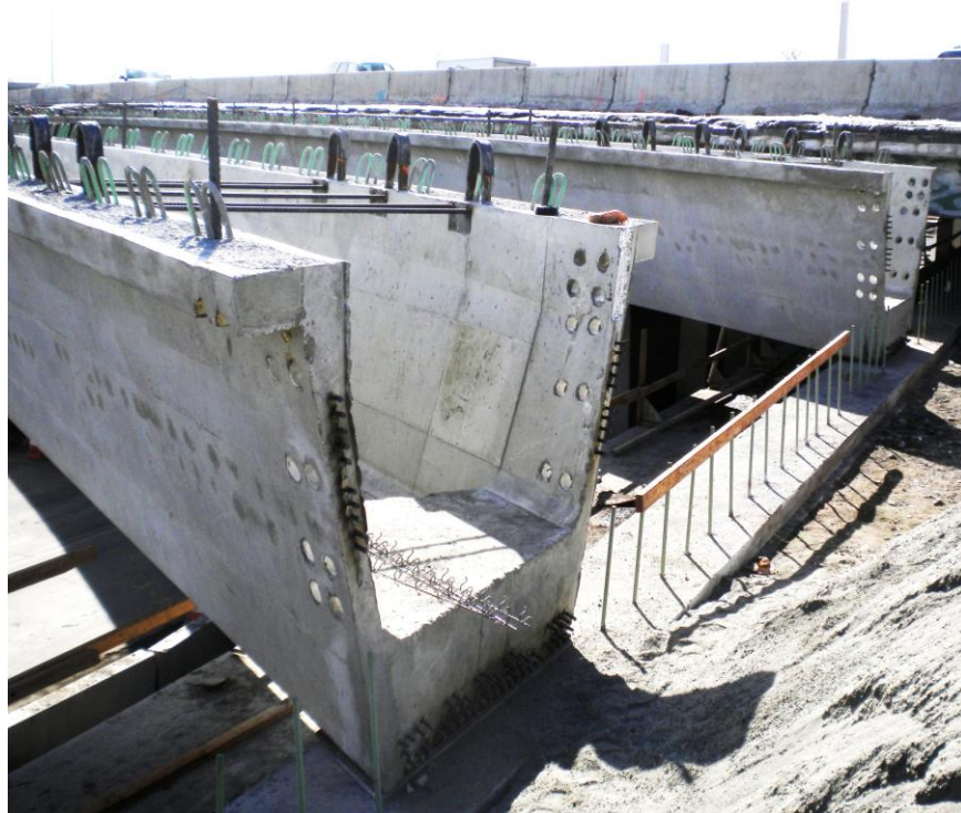
Fig. 15: U72 Precast Girders on Abutment Cap
