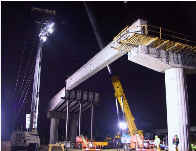
Figure 11 – Setting the First Girder Segment E
