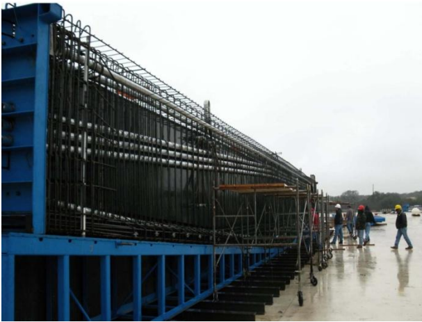
Figure 9 – Variable Depth B & D Girder Segment Casting
