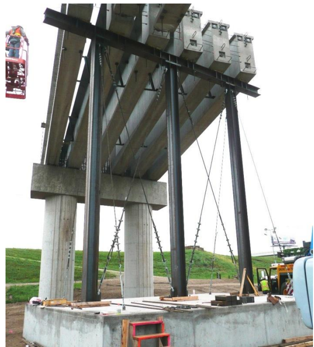
Figure 6 – Temporary Support Tower and Tie-Down
