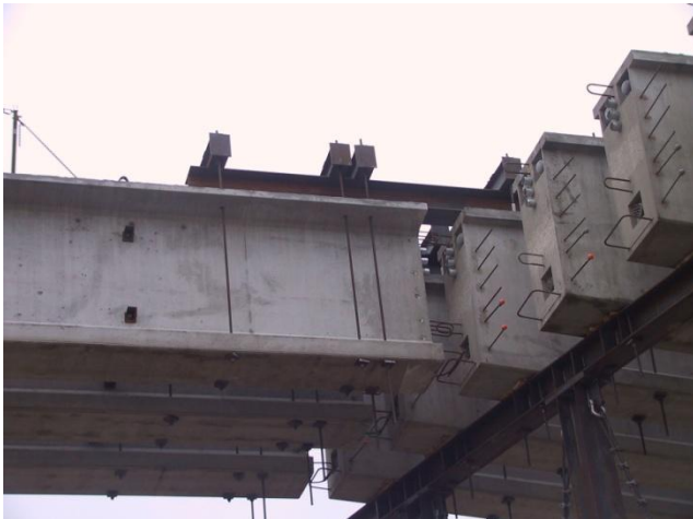
Figure 7 – Girder Strong-Back Beams
