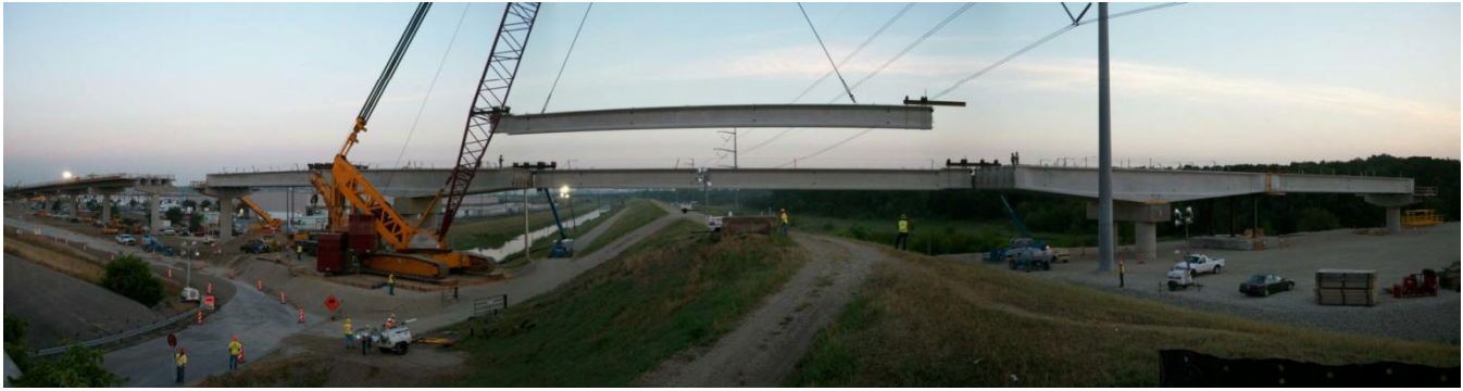
Figure 12 – Erecting Girder Segment C
