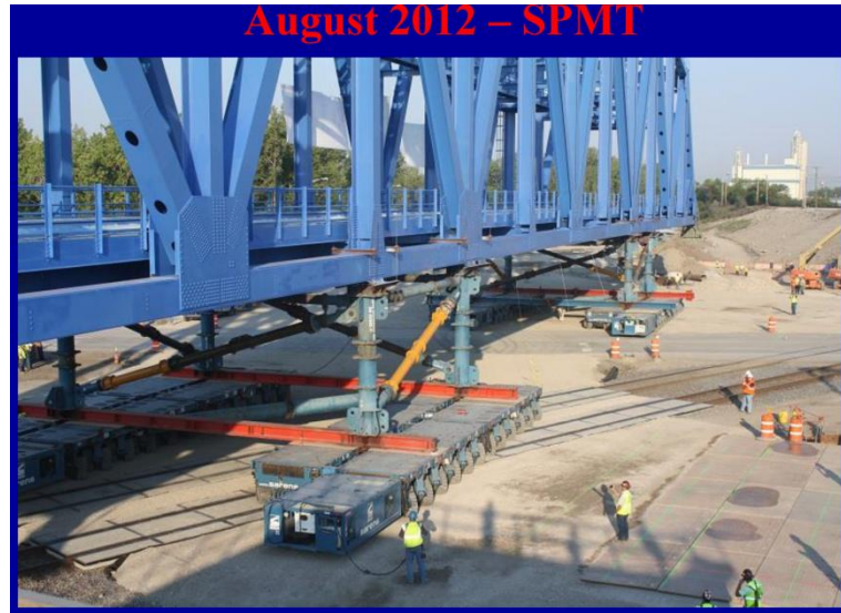
Fig. 3 SPMT Set Up (CDOT)
