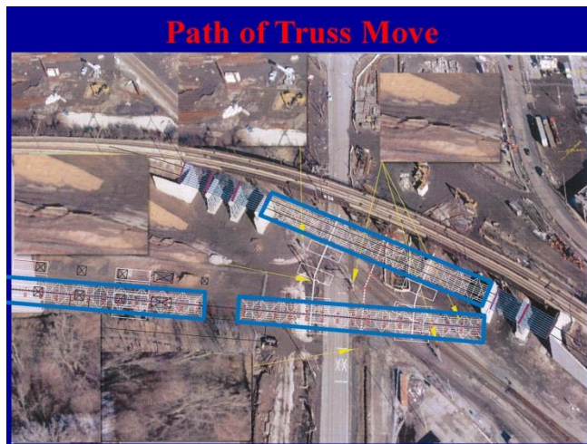
Fig. 2 Path of Truss Movement (Chicago Department of Transportation)
