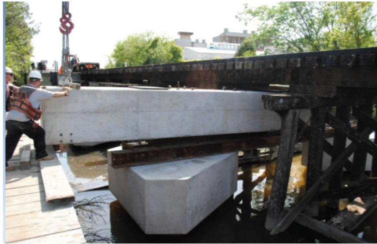
Fig. 10 Precast Pier Cap Installation (AREMA)
