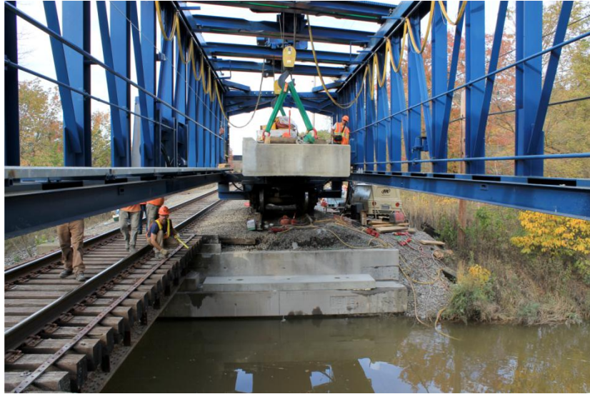
Fig. 12 Precast Bridge Slab Installation (AREMA)
