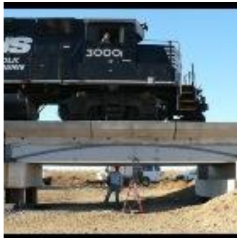
Fig. 15 First HCB Railroad Bridge (HC Bridge Company)
