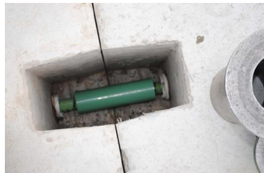
(b) Post-tensioning bar splicer
