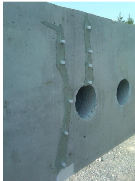
(b) Repaired crack
