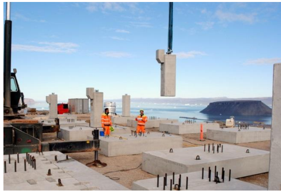
Figure 7 – Installing a building pier
