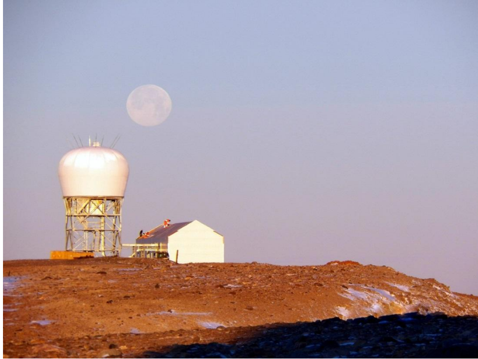
Figure 14 – Contractor installing roofing material at the end of the construction season
