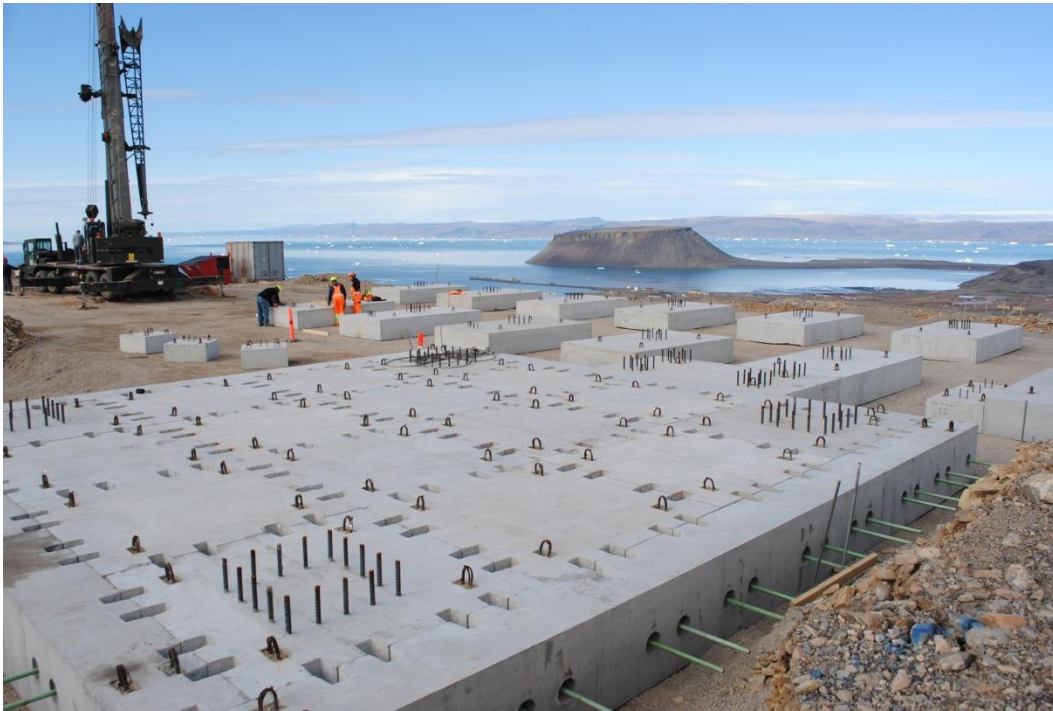
Figure 10 – Foundation placement
