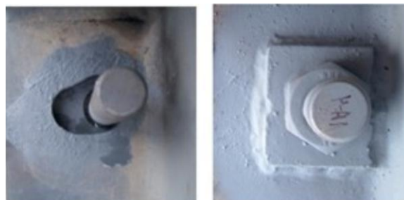
Figure 8 – Modified Anchor Rod Connection
