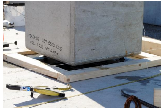
(b) Placing pier with splice sleeves onto footing dowels
