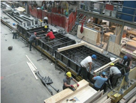
(a) Preparing footings in forms
