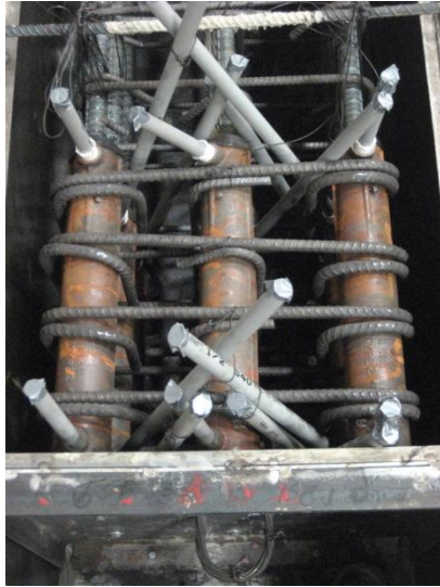
(a) Splice sleeves in pier form
