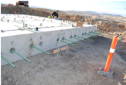
(a) Post-tensioning bar stub
