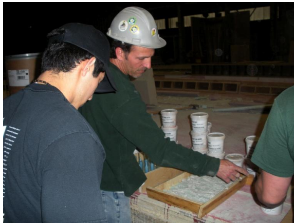
Fig. 4 Precast foreman suggesting additional reinforcement for student's formwork prior to casting.
