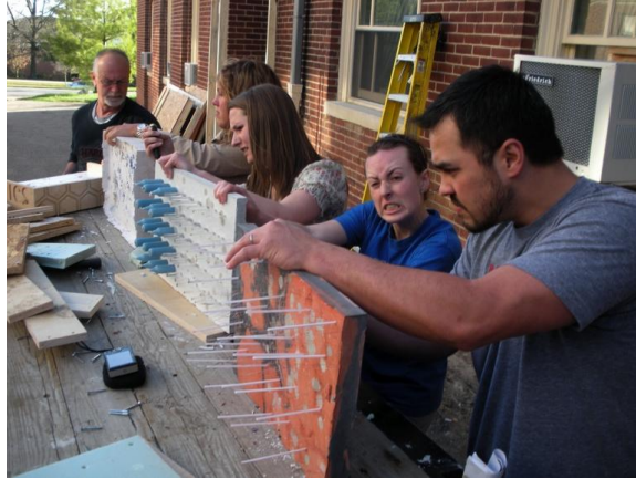
Fig.7 Stripping formwork is not as easy as it looks.
