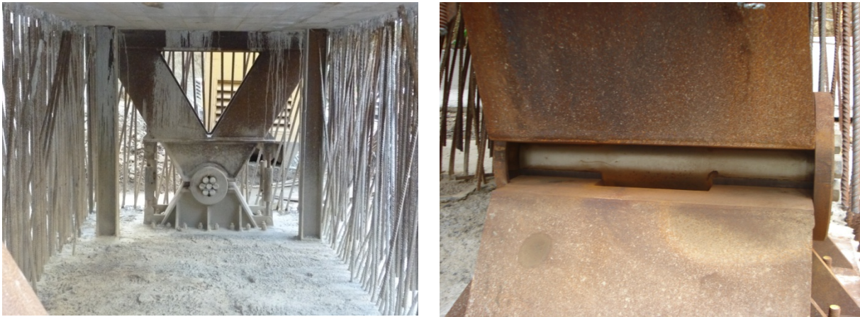
Fig. 8. Lateral view and detail of hinges
