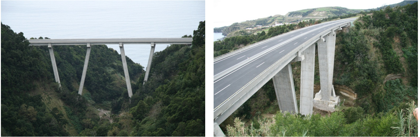
Figure 15. Overall view of the bridge
