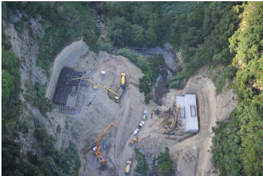
Fig. 4. Aerial view of the construction of foundations
