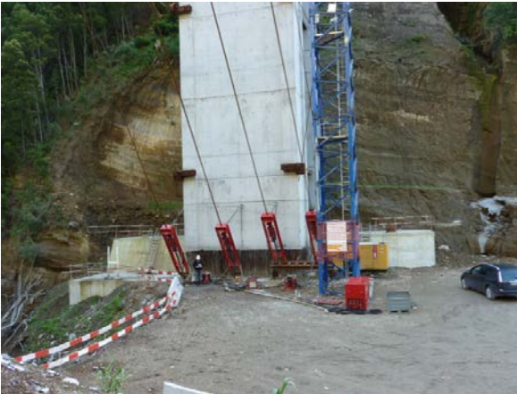
Fig. 7. Lifting units arrangement for pile caps and hammerheads
