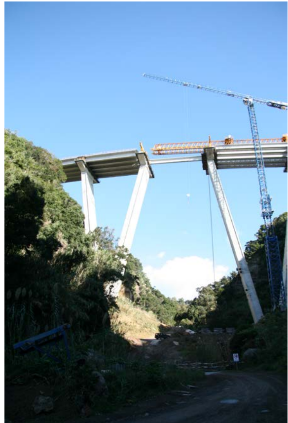
Figure 13. Central spine beam at middle span
