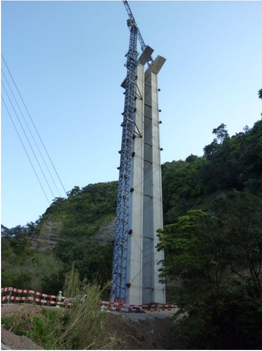
Fig. 5. Temporary bracing
