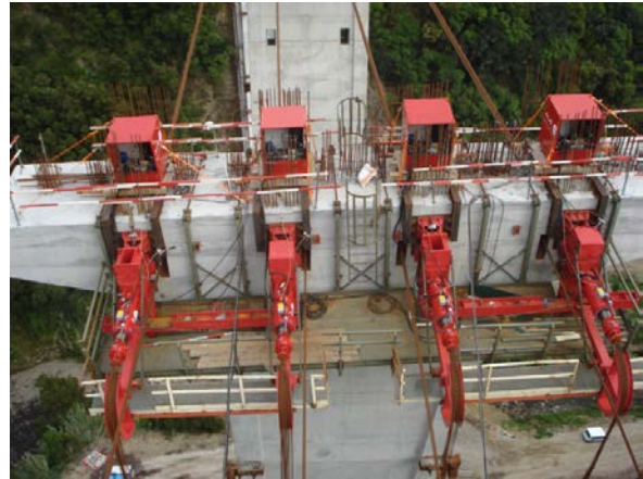
Fig. 7. Lifting units arrangement for pile caps and hammerheads
