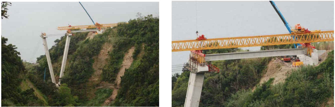
Figure 12. Launching of the first viaduct girder. View from upstream.
