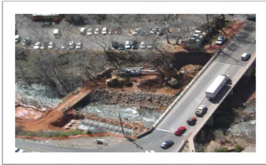
Fig. 2: Existing Bridge and Temporary River Crossing
