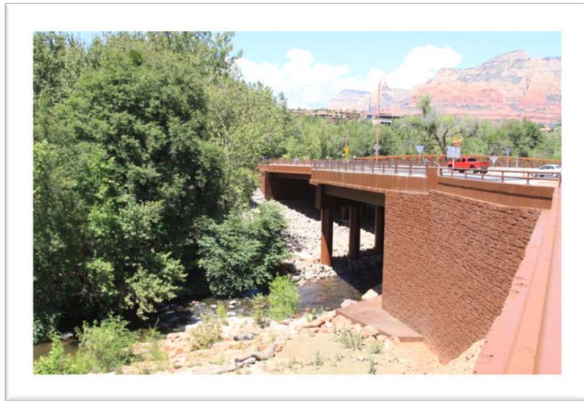
Fig. 16: Final Oak Creek Bridge
