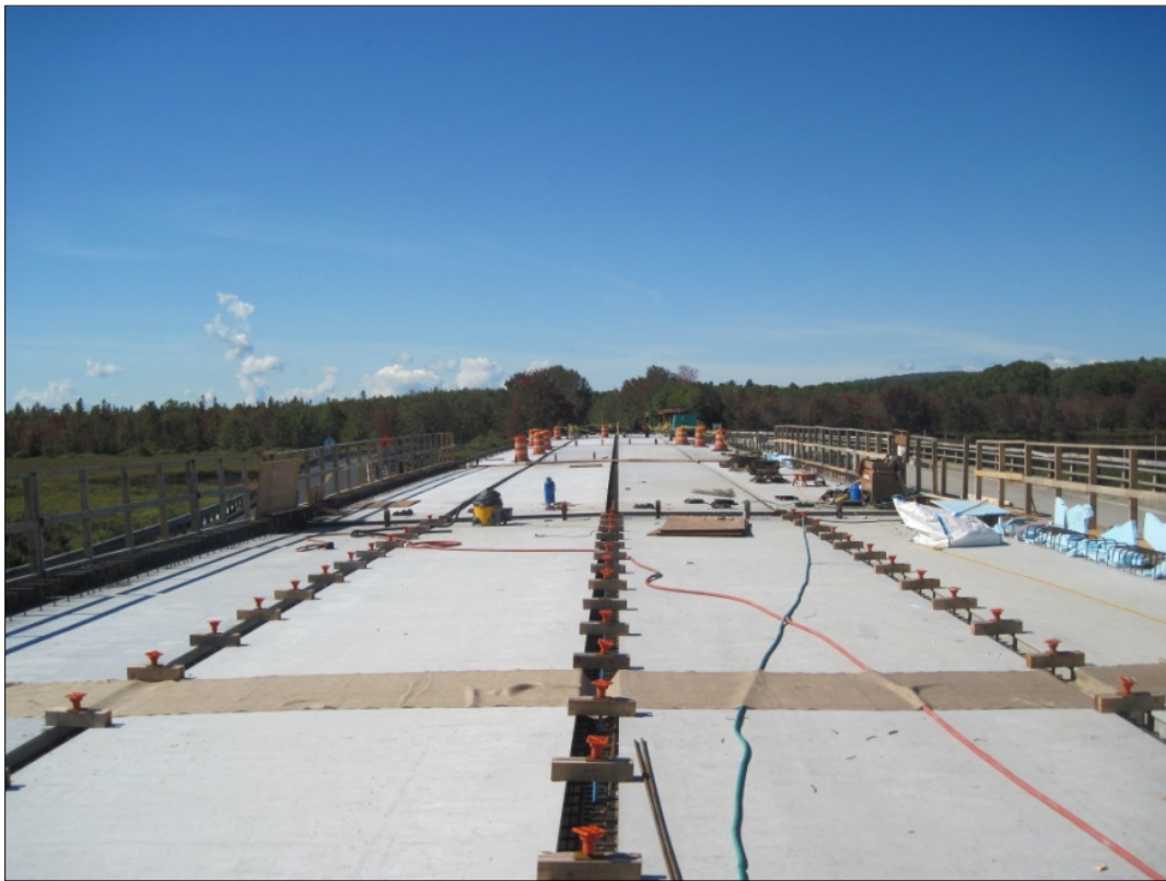
Fig. 23 Longitudinal closure joints
