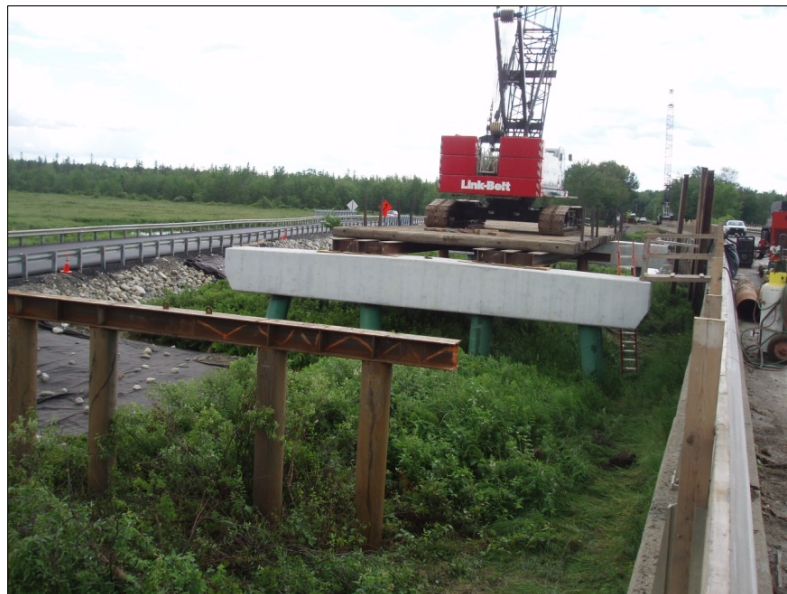
Fig. 16 Pile driving operation with temporary bent in foreground
