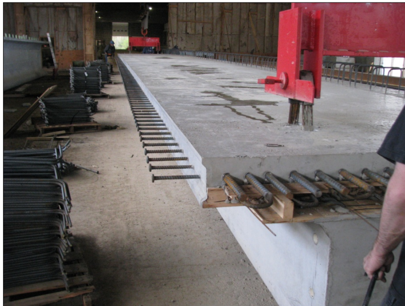
Fig. 13 Completed NEXT D beam
