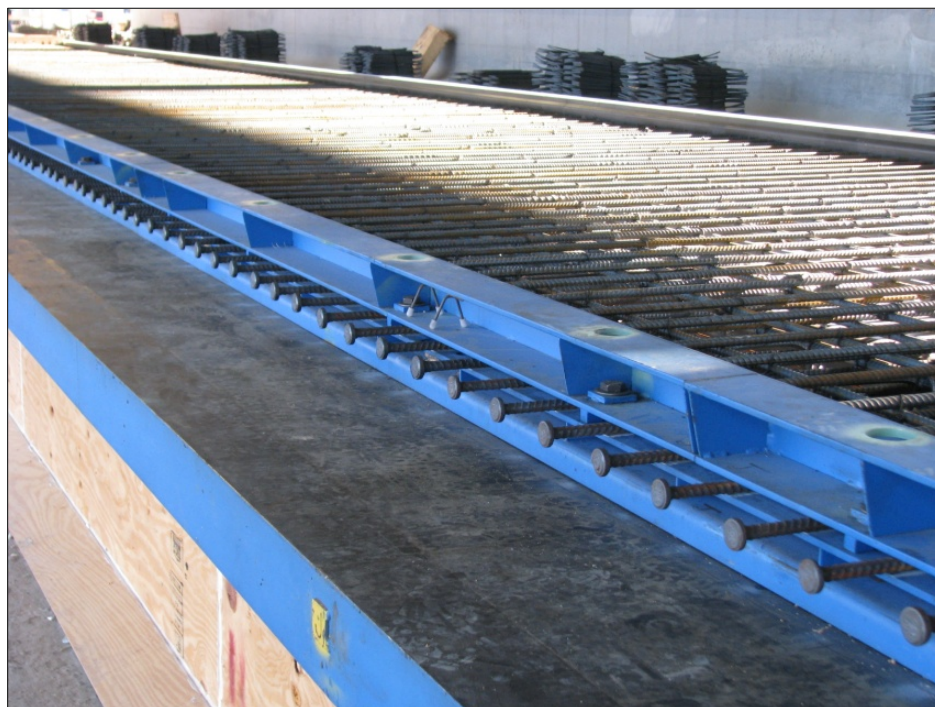
Fig. 11 NEXT D beam with steel studs
