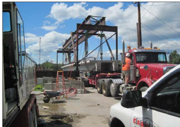
Fig. 19 NEXT beam positioned under gantry crane
