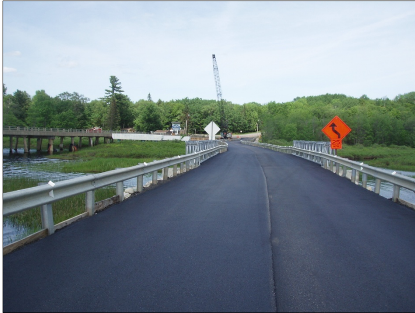
Fig. 5 Temporary detour roadway and bridge
