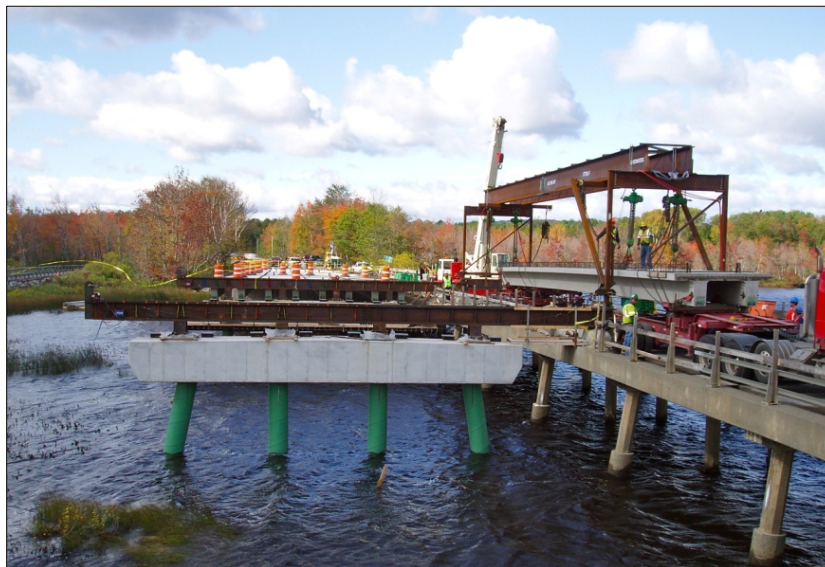
Fig. 6 Erection setup
