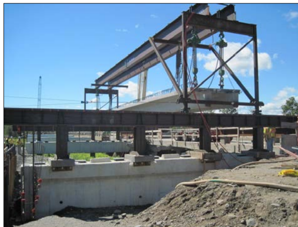
Fig. 22 Gantry crane moving laterally to place NEXT beam
