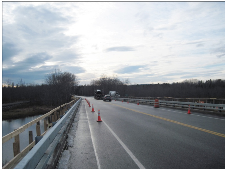
Fig. 2 Bridge open to traffic
