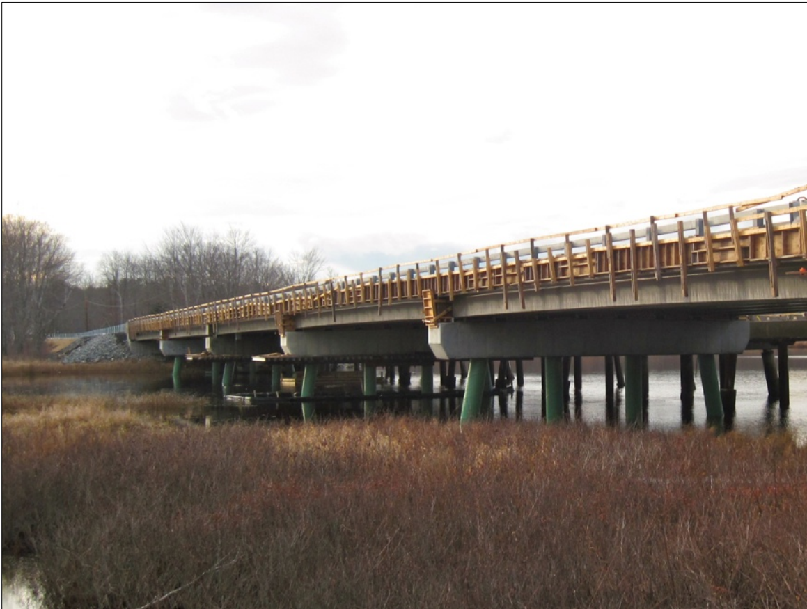
Fig. 14 Elevation view of several pier bents
