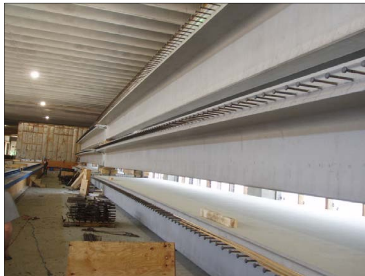
Fig. 25 NEXT beams stored at precaster
