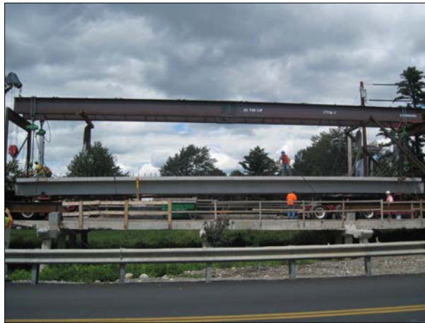
Fig. 21 NEXT beam lifted off truck
