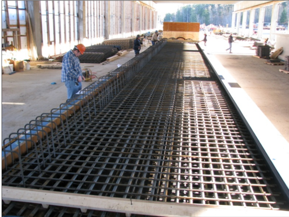
Fig. 10 NEXT D beam in casting bed
