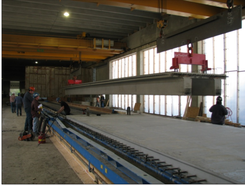
Fig. 12 NEXT D beam lifted from casting bed
