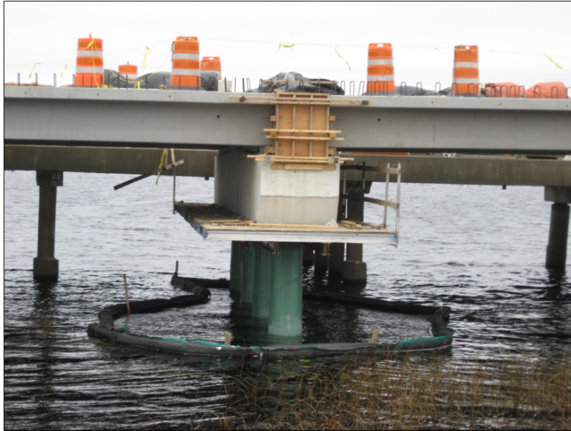
Fig. 15 Elevation view of fixed pier bents
