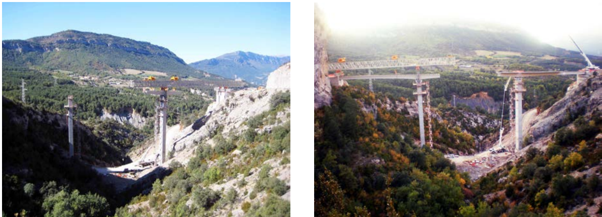
Figures 27 and 28: “La Espluga” bridge during construction (2011).
