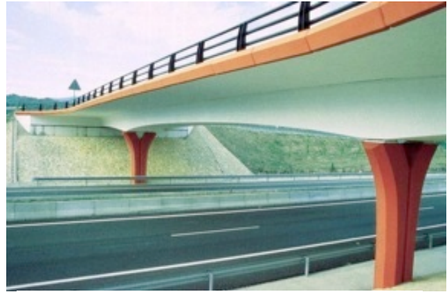
Figure 1: Typical three-span crossing, with parabolic variable depth.
