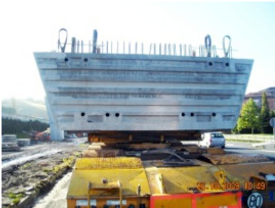
Figures 15 and 16: Diaphragm and Cross-section of a joint between U girders.
