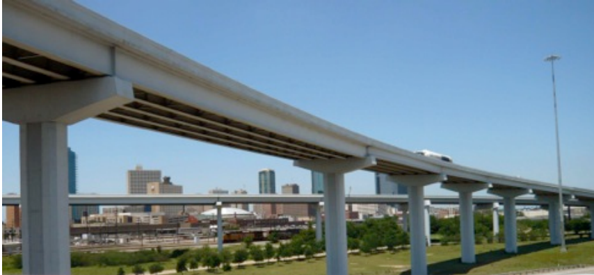
Figure 18: Typical elevated highway, on the outskirts of Dallas.
