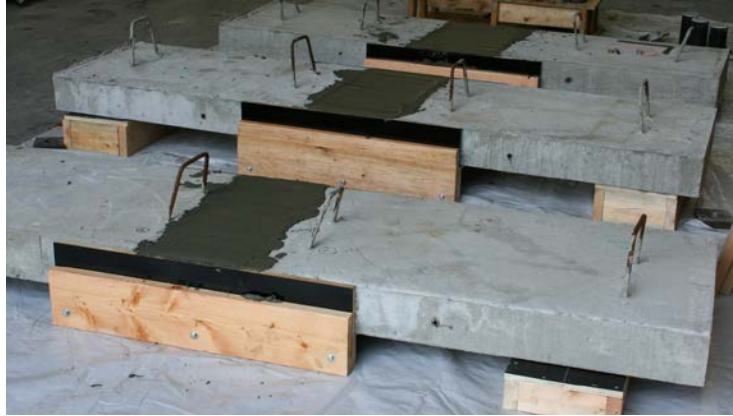
Fig. 1 Casting of deck-level connection specimens: Non-shrink grout connections with 8", 12" and 15" non-contact bar laps are shown.
