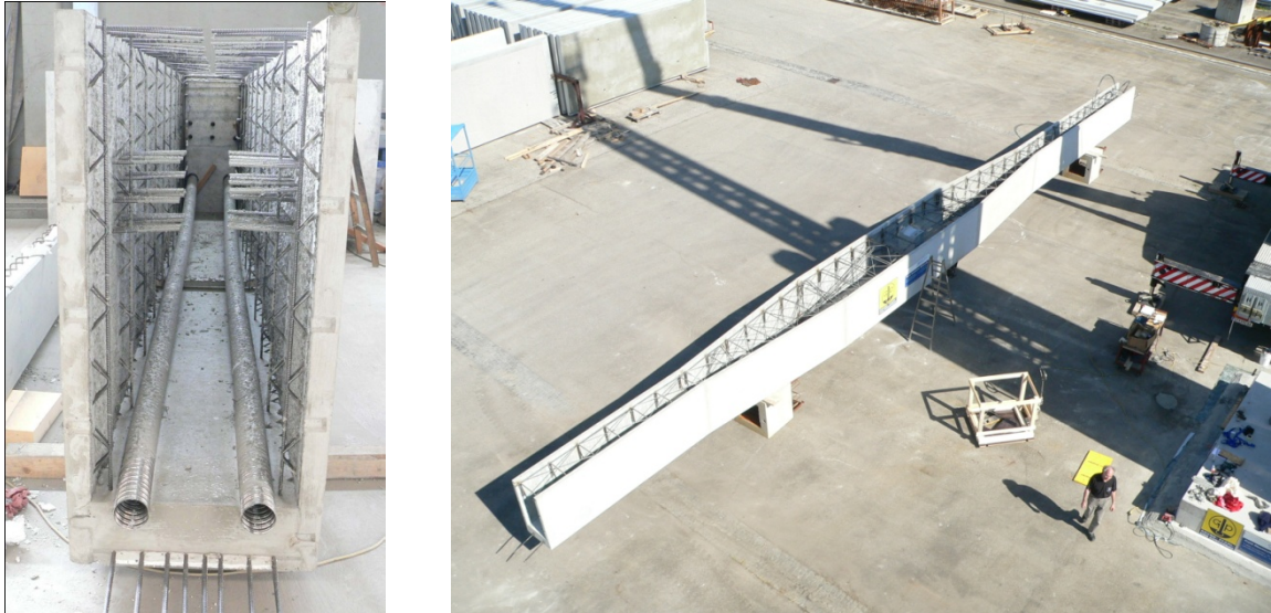
Fig. 9 U-shaped concrete bridge girder
