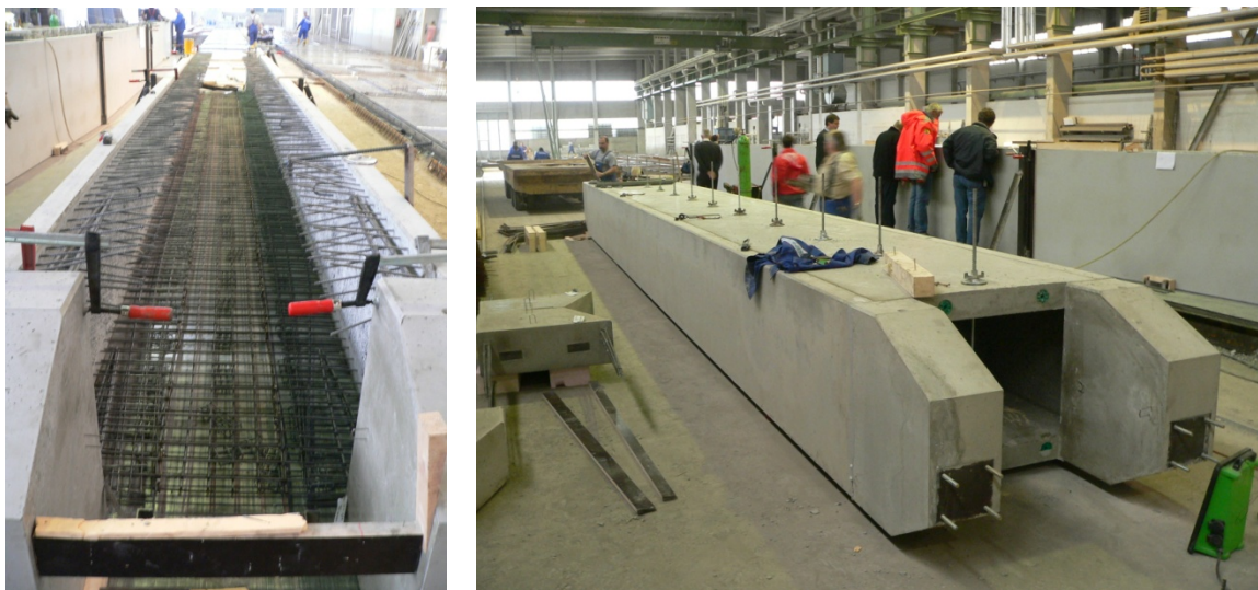
Fig. 10 Prefabrication of the compression struts
