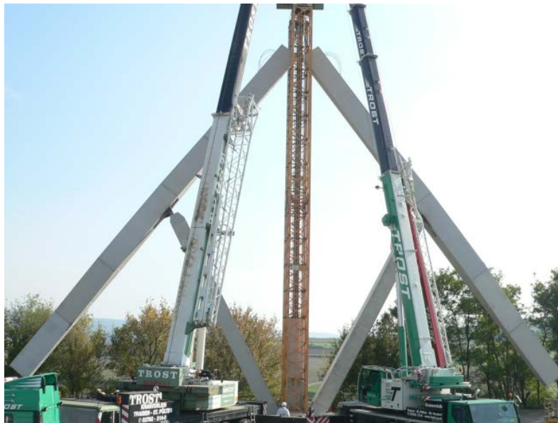
Fig. 12 Lowering operation of bridge girders
