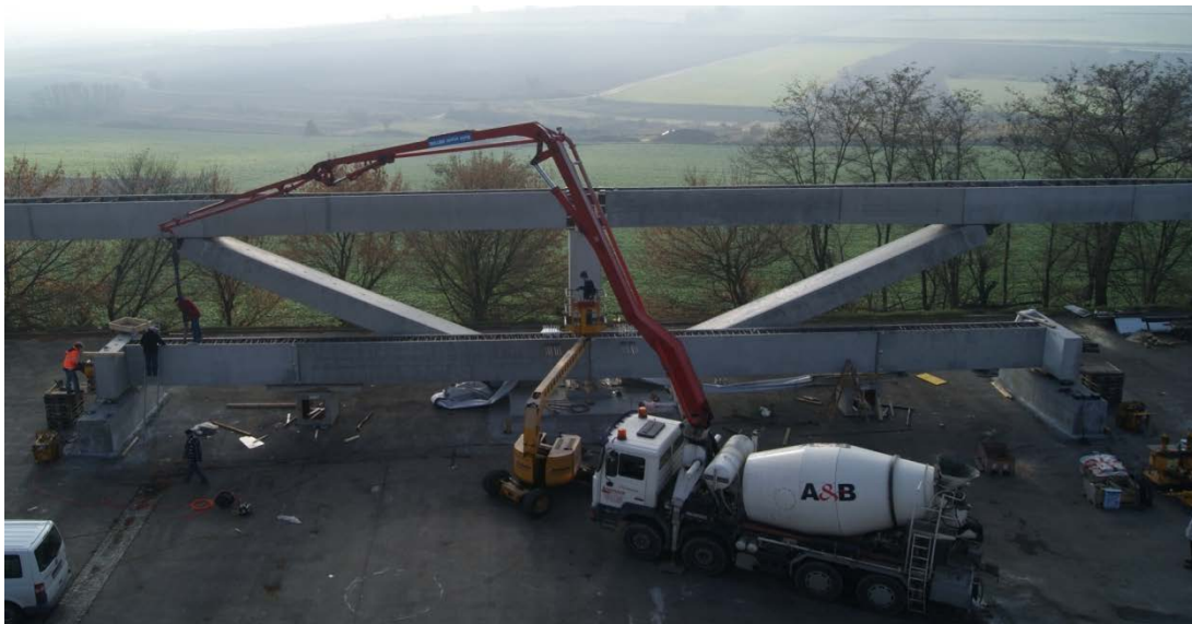
Fig. 14 Erection of a 30 m single-span girder without falsework
