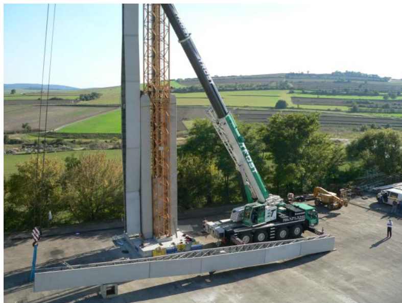
Fig. 11 Lifting of bridge girders
