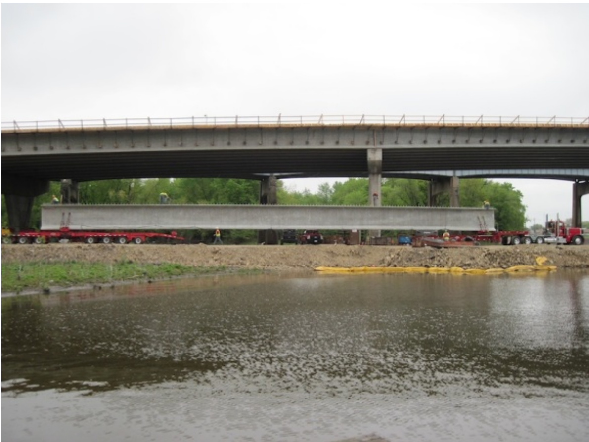
Fig. 13: 96MW Beam at Hastings Bridge Site 11
