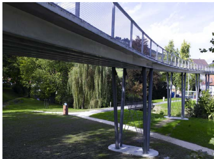
Fig. 1 Pedestrian Bridge with TRC superstructure in Albstadt, Germany
