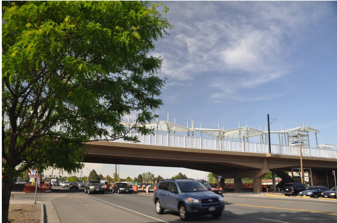
Fig. 1: LRT Bridge and Station over Wadsworth Boulevard
