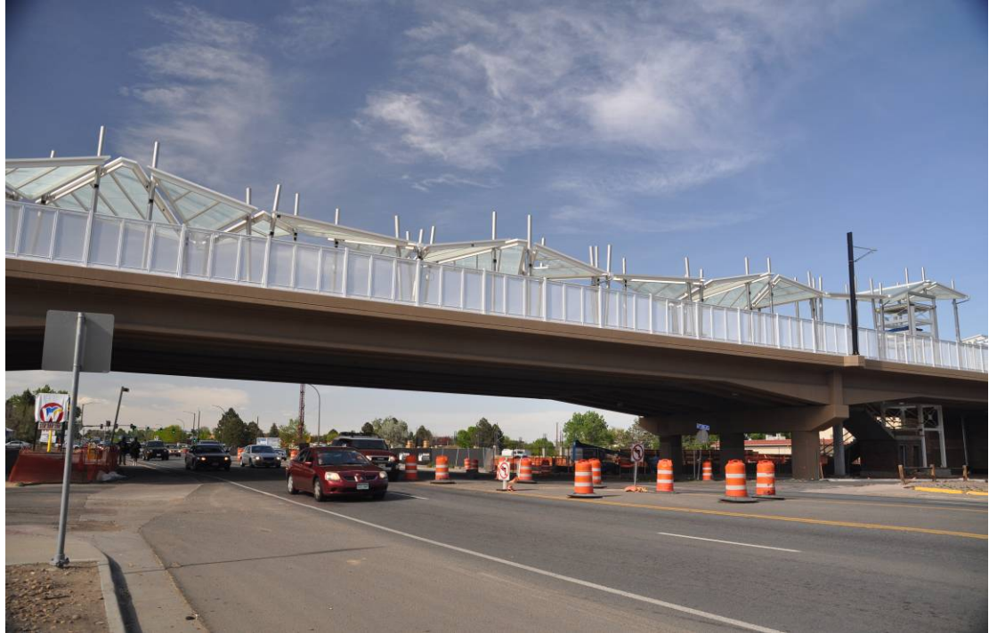
Fig. 15: Final Bridge and Station Construction, April 2012
