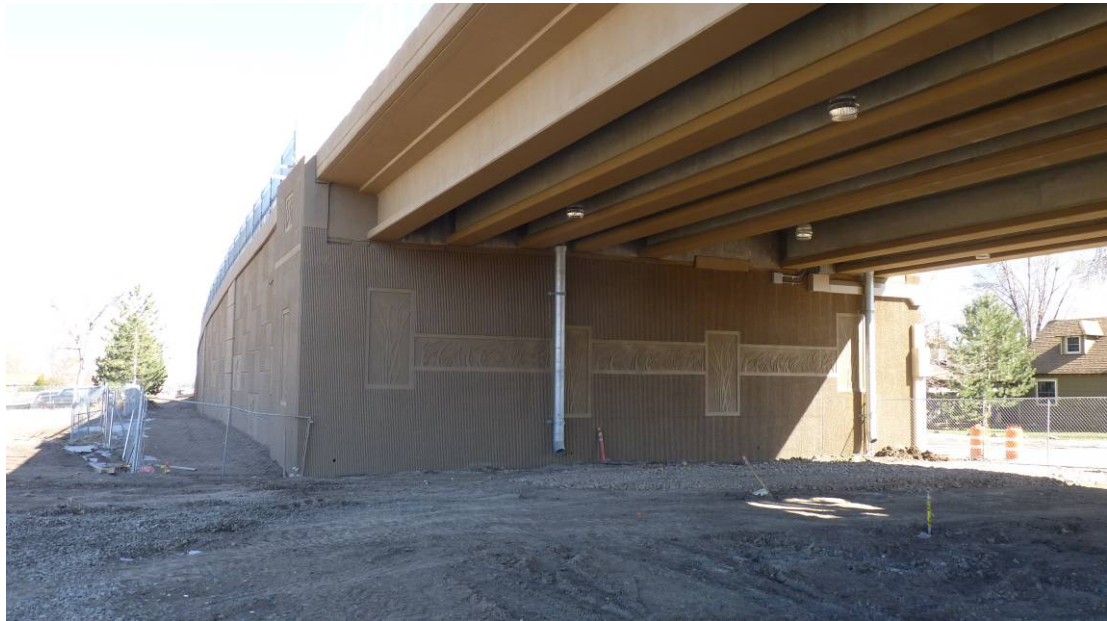
Fig. 7: East Abutment and MSE Header Bank Approach
