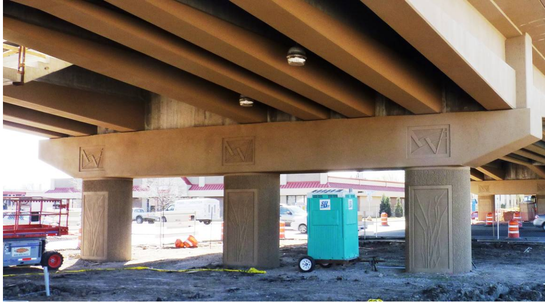
Fig. 9: Completed Bridge at Interior Bent
