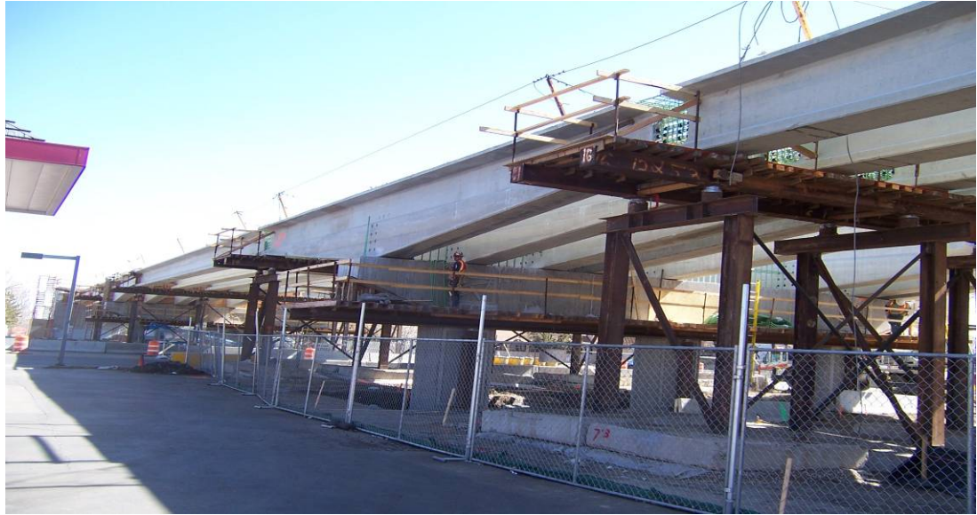
Fig. 14: Precast Girders on Temporary Falsework Towers
