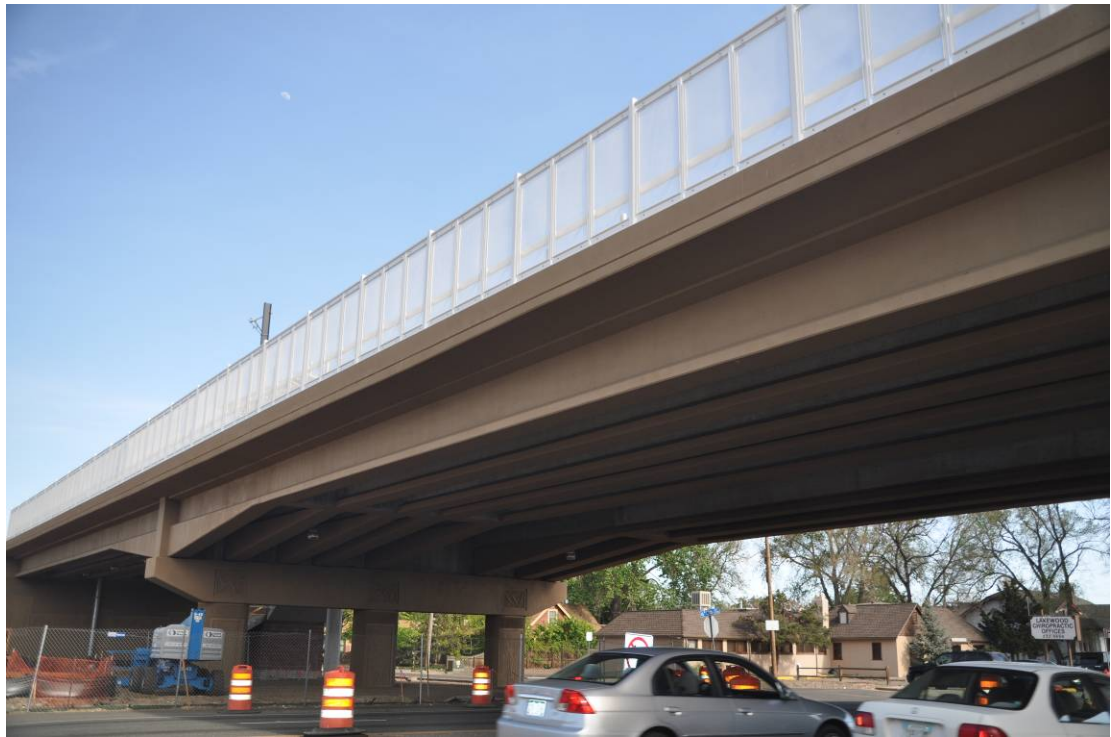
Fig. 4: Completed LRT Bridge over Wadsworth Boulevard
