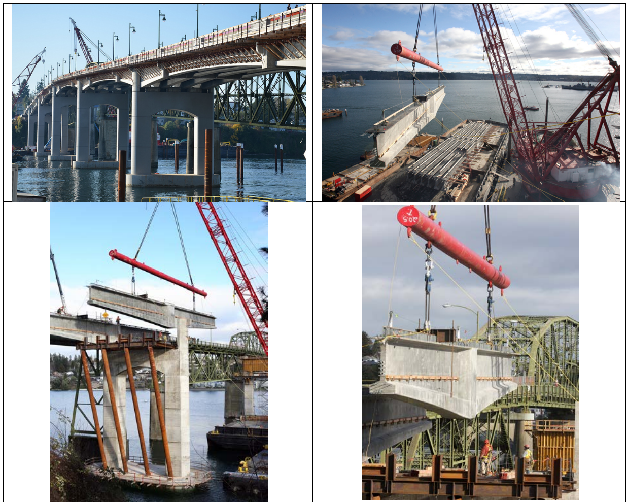
Fig. 1 shows the construction of or the Manette Bridge in Bremerton, WA
