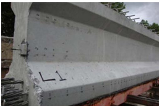
Figure 13 - DEMEC Points at the end of the Specimen
