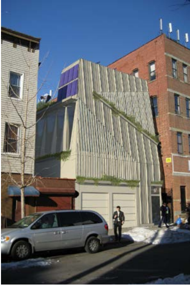
Figure 28: Preliminary rendering for proposed precast building at 97 Sutton Street, Brooklyn, New York. The building has two residential units built above a single-story garage. Note the vertical fins to mitigate eastern sun for adequate day lighting.
