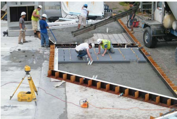
Figure 23: Roof panels being formed with students of the New Jersey Institute of Technology, July 2011.
