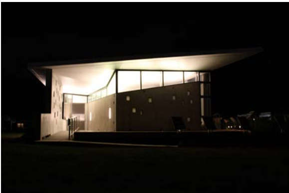
Figure 26: View looking east at night of the completed eNJoy! House in West Potomac Park, Washington, DC, September 2011. Note the use of clerestory windows gives the impression that the heavy, cantilevered precast roof is floating above the house.
