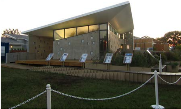
Figure 12: eNJoy! House; New Jersey Institute of Technology and Rutgers University – 2011 US Department of Energy Solar Decathlon competition
