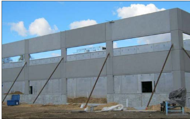
Figure 1: Precast walls with large openings: truck entrance (top); parking structure (bottom)
