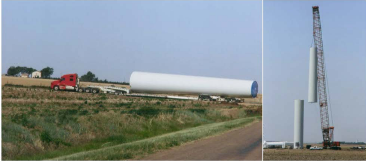
Figure 3: Transportation and erection of complete steel tube segments 6 .
